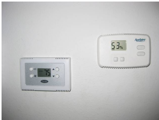
PHA houses: Aprilaire model 70 dehumidistat installed adjacent to the thermostat in the main living area
