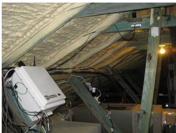
Weather-tight enclosure fastened to roof truss
