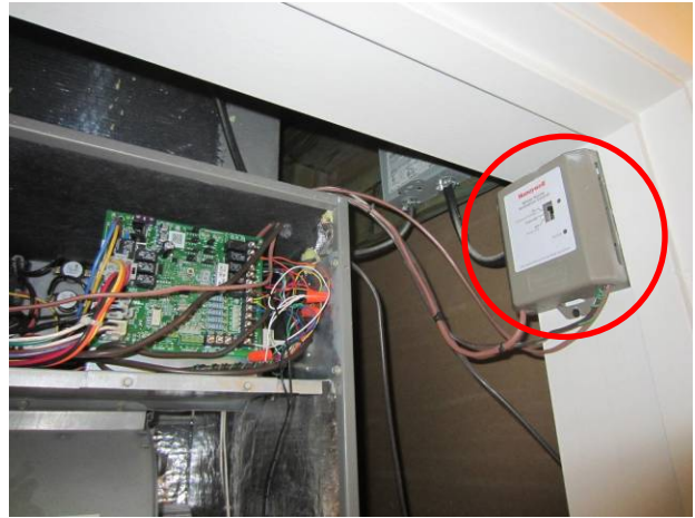
BDC houses: Honeywell W8150 ventilation control installed on the inside of the door
