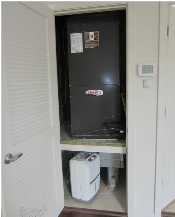
HVAC system located in a mechanical closet in the main living space. Note louvered door for return airflow.
