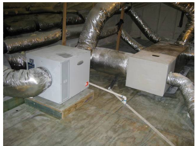
Another photograph, showing condensate line from dehumidifier
