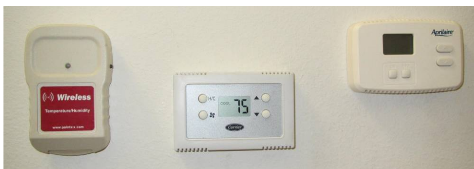
Figure 16. Wireless T&RH sensor wall mounted near the thermostat and Aprilaire model 70 dehumidistat
