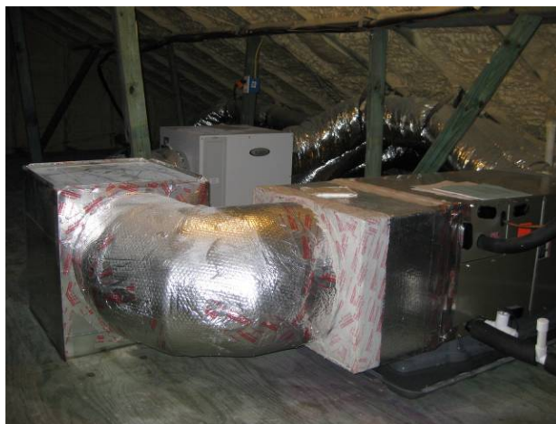
HVAC system and dehumidifier located in unvented cathedralized attic
