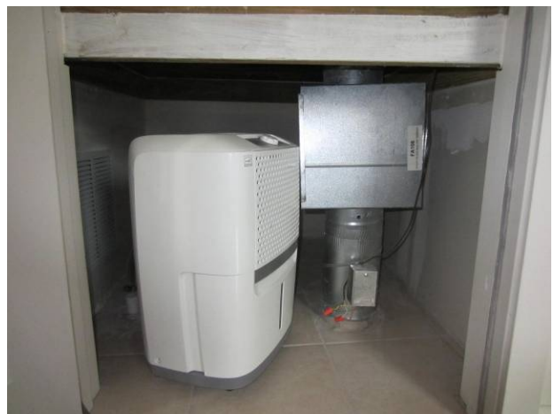
Close-up of open return with standalone dehumidifier and outside air duct. Note the filter/manual damper box and the motorized damper underneath.
