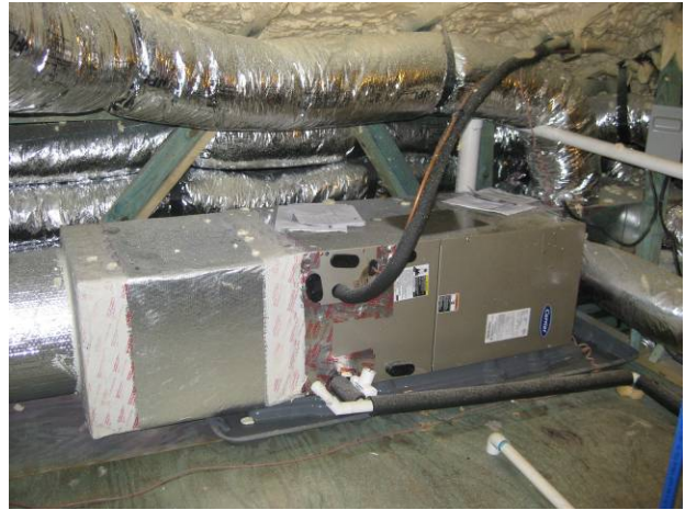
Closer photograph of horizontally oriented air handler
