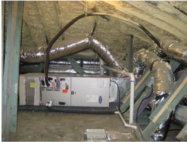
HVAC system located in unvented cathedralized attic
