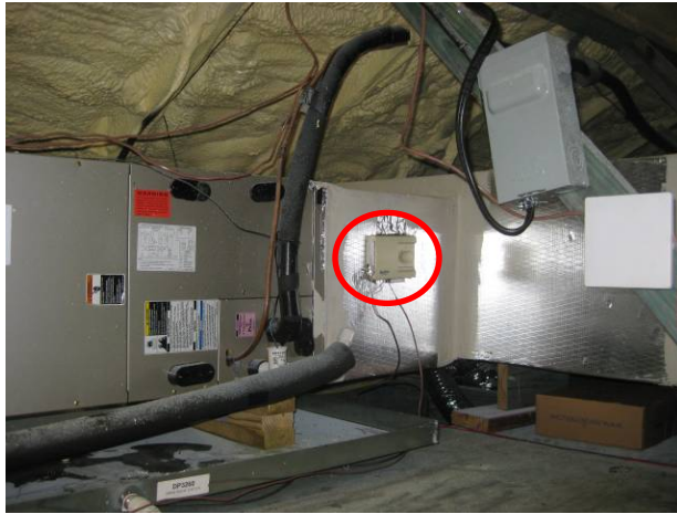
PHA houses: Aprilaire 8120 ventilation control installed on the return plenum
