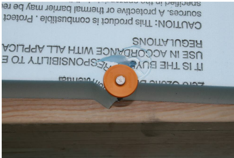
Figure 23. Nail pulling through XPS
