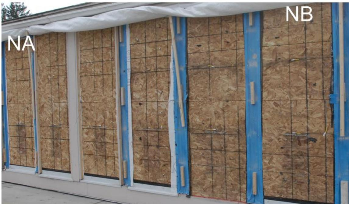
**Figure 47. Exterior OSB sheathing on the north orientation immediately following deconstruction (photo taken from the opposite direction of Figure 46)**
