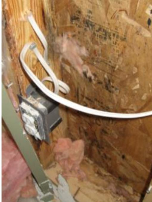
**Figure 39. Example of air leakage condensation durability issues**
