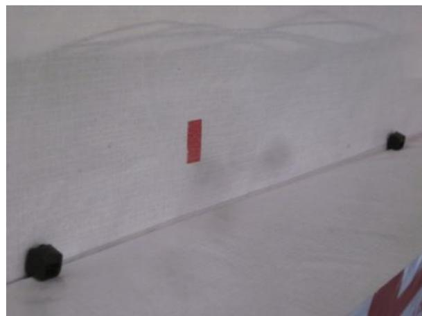
**Figure 11. Spacers installed in top of drainage gap**
