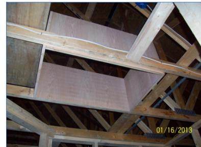
**Figure 28. Insulation dam at attic access**
