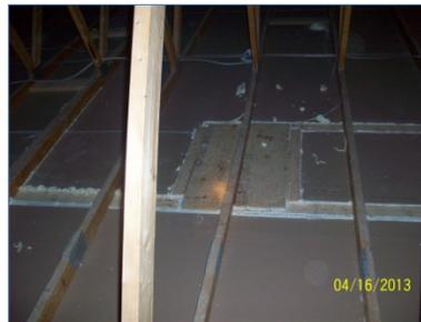
**Figure 27. Sealed air barrier at the HVAC duct chase**
