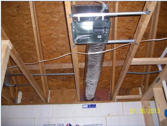
**Figure 31. Short and direct bath exhaust fan duct**
