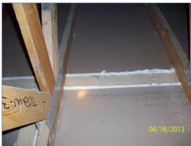
**Figure 26. Sealed top plate**
