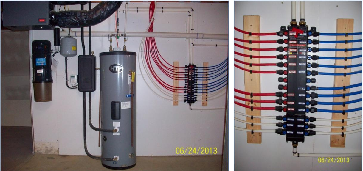
**Figure 29. Solar hot water storage tank and PEX piping manifold**
