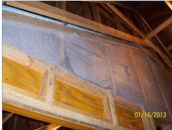
**Figure 25. Knee wall insulation**
