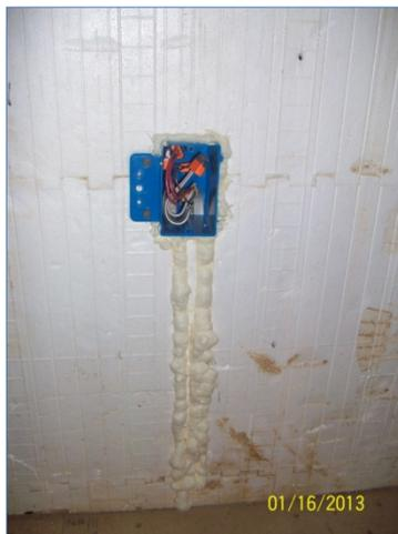
**Figure 19. Foam over rough wiring at ICF**
