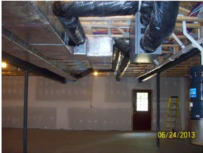
Figure 7. Duct system Installed in basement
