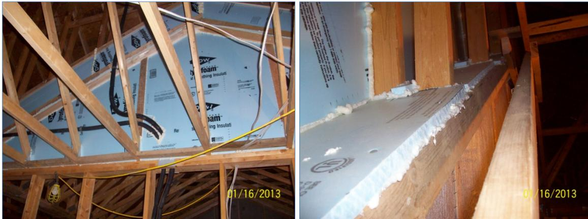
**Figure 24. Knee wall air barrier**
