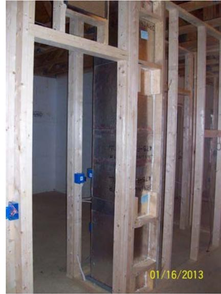
Figure 8. Simplified central return inside framed duct chase
