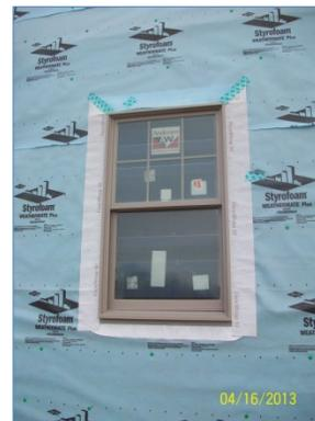
**Figure 17. Window flashing**
