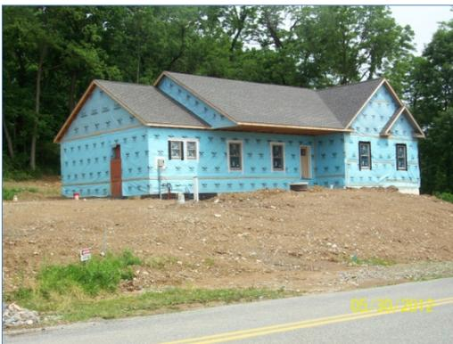
**Figure 16. House wrap installed before summer break**
