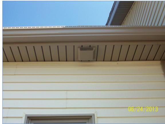
**Figure 32. Bath exhaust duct termination at soffit**
