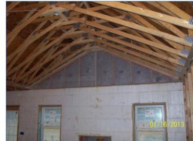
**Figure 23. Framed gable after air sealing and insulation**
