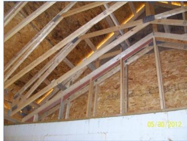
**Figure 22. Framed gable before air sealing and insulation**
