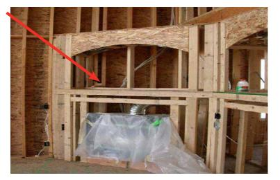
Fireplaces are often installed against open framing without a proper air barrier or insulation. The arrow points to the framed exterior wall where insulation and an air barrier should be installed (Source: EnergyLogic).
