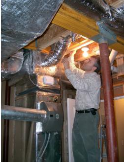
(*Top*) Mastic is a thick, gooey substance that is painted onto seams and joints. Duct seams and joints should be sealed with mastic or approved metal tape, not duct tape (Photo Source: FSEC).
