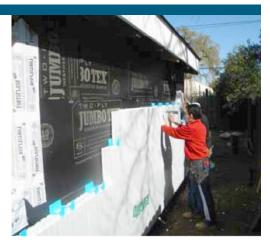
**Exterior foam block insulation.** These blocks stack up like bricks. The insulation shown provides an R-value of 18 (Photo Source: DOE).
