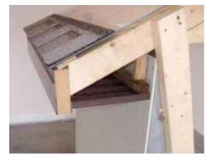
The fascia was redesigned to extend 1 inch below the soffit to form a drip edge, directing water down and away from the house.
