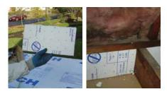
Figure 4. Air seal floor joist cavities under kneewalls by filling the cavities with rigid foam insulation, OSB, or another rigid material that is cut to fit and sealed at the edges with caulk (as shown here and below). Another option is to block the joist cavity with fiberglass batts that are rolled and stuffed in plastic bags or covered with spray foam.
