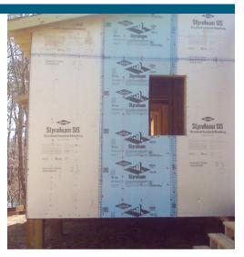
**Exterior rigid foam.** Rigid foam insulation is installed on the exterior of a new framed home in Georgia. The rigid foam takes the place of OSB wall sheathing (Photo Source: IBACOS).
