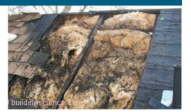
Moldy fiberglass batts. The fiberglass insulation in this unvented cathedral ceiling absorbed moisture, leading to mold and wood damage. Building America scientists do not recommend using fiberglass or cellulose in a cathedral ceiling or flat roof, unless rigid or spray foam insulation is installed above the fiber to form an air and moisture barrier (Photo source: BSC).
