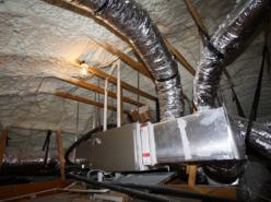
(*Top*) **Spray foam insulation.** Spray foam was used to simultaneously air seal and insulate this ventilated attic. Baffles installed in each rafter bay keep the insulation from blocking the soffit vents (Photo Source: WSU Energy Office).
