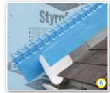
Installing Sidewall and Kick-out Diverter Flashing on Homes with Housewrap over OSB or Plywood Sheathing
