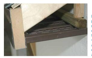
Perforated soffit board product with recessed rather than surface openings was installed to limit water intrusion while encouraging greater air circulation and faster drying within the eave assembly.
