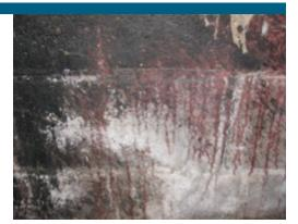
Wet masonry. Avoid insulation strategies that increase moisture retention in masonry walls. Wet masonry can develop mold and efflorescence, a chalky salt residue (Photo Source: PNNL).
