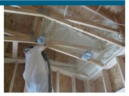
**Polyurethane foam insulation**. Leave the installation of spray foam to trained professionals. Toxic gases emitted during application are hazardous to skin, eyes, and lungs (Photo Source: NAHB).
