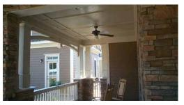
If the cantilevered floor over this porch isn't properly air sealed and insulated, the room above will feel cold and drafty in the wintertime (Photo Source: Pine Mountain Builders).
