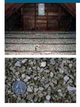
Vermiculite insulation. If you have vermiculite insulation in your attic or walls, you should assume that it contains asbestos and be careful to avoid exposure. Vermiculite was commonly used before 1990 (Photo Source: EPA).
