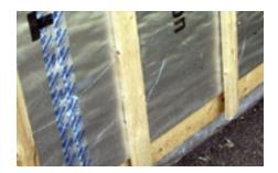
Air barrier. The new wall assembly has foilfaced rigid foam sheathing, carefully taped to provide a continuous air barrier. Furring strips in front of the foam create an air space for proper drainage.
