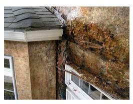
Improper flashing can allow rain water into walls, causing significant damage (Source: DryFlekt Products, Inc).
