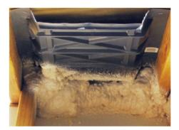
Figure 5.5. Baffles. Your contractor will install vent baffles to maintain a 2-inch continuous ventilation channel above the insulation. Continuous ridge vent ridge vent Attic insulation Attic ventilation 2 inch minimum space Insulation vent baffle Continuous soffit vent
