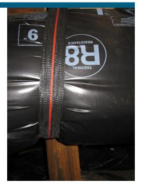
All ducts should be laid straight and adequately supported. Flex ducts should be stretched tightly; loose, sagging ducts can greatly restrict air flow (Photo Source: PNNL).
