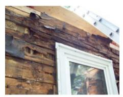
**Rotting wood**. Hidden under the vinyl siding was the home's original wood siding, which was moldy and rotten. A poorly designed wall assembly had allowed water to penetrate for years.
