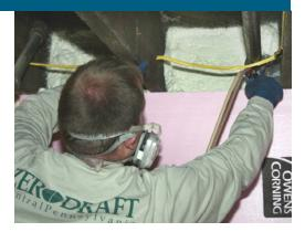
**Basement wall insulation**. In this Pennsylvania basement, rigid XPS foam insulation is attached directly to the concrete basement walls with spray foam. Rim joists are insulated with spray foam. Frame walls will be built to finish the basement (Photo Source: Asdal Construction).
