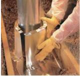
You can make a sheet metal or gypsum board dam to keep insulation from touching hot metal or masonry chimneys and flues (Source: EPA 2008a).
