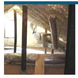
**Unvented attic**. This attic has been sealed and insulated with spray foam insulation applied under the roof deck. This turns the attic into a conditioned space for HVAC equipment (Photo Source: W. Hawthorne).
