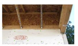
The house wall separating the porch attic from the rest of the house was correctly air sealed in this new home to prevent air from flowing into the home and causing heat loss.
