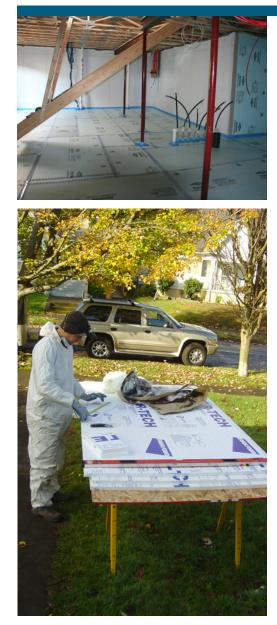
(*Top*) **Interior rigid foam insulation**. Rigid foam has been installed on the interior basement walls of this new home in Pennsylvania. The ground has also been covered with rigid foam, in preparation for pouring the concrete floor slab (Photo Source: IBACOS).
