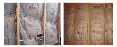
*(Left)* **Poorly installed batts.** These fiberglass batts have reduced R-value because of the gaps and compressed areas (Photo Source: PNNL).
