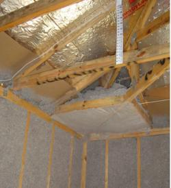
(*Top*) **Dense-pack fiberglass**. In this newly built home, dense-pack fiberglass is held in place with netting. This is a popular choice for retrofit insulation, blown into open cavities or installed using the drill-and-fill method (Photo Source: Bob Ward Company).
