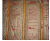
Faced fiberglass batt insulation
