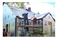
**Exterior insulation**. Workers installed a continuous air barrier on the above-grade portions of the house, including the roof, then wrapped it again with continuous layers of insulation.
