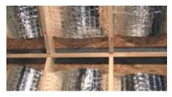
In hot climates, radiant barriers can cut cooling costs 8% to 12%. In this house, a flexible radiant barrier material was draped over the rafters before installation of the roof deck. The material also can be stapled to rafters from the underside (Photo Source: Universal Forest Products).
