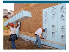
**Exterior insulation**. At this new home, in Pittsburgh, workers install rigid insulation on the foundation and exterior walls. Rigid foam insulation can be installed on the walls of existing homes when the siding is removed. Insulating the foundation of an existing home is more difficult; it requires digging a trench down to the frost line (Photo Source: IBACOS).
