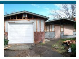
**Opportunity to insulate**. The siding needed to be replaced in this major renovation of an uninsulated Sacramento home. Removing the siding created an opportunity to add rigid foam insulation to the exterior of the walls (Photo source: SMUD).
