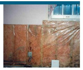
Vapor retarders and mold. Vapor barriers like this polyethylene sheet can trap moisture in walls. The damp fiber insulation in this wall developed mold and odors (Source: BSC).
