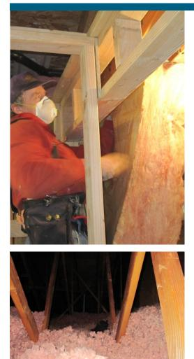
Fiberglass. Take care when handling fiberglass insulation, which can irritate skin and lungs. Keep kraft facing on batts away from hot fixtures. Install vent baffles to keep loose-fill insulation from blocking attic vents. Blocked vents can lead to problems with moisture, mold, and wood rot (Photo Source: PNNL).
