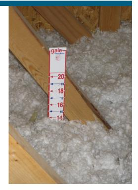
**Depth of insulation**. When installing loose-fill insulation in an attic, your contractor should staple rulers in several places to ensure the insulation is deep enough and has been spread evenly. These rulers are also useful for measuring changes over time as insulation settles (Photo Source: PNNL).
