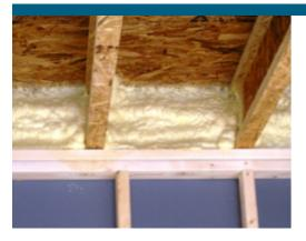
**Insulated rim joist.** Stop air leakage through the rim (or band) joist at the top of the basement wall with spray foam (shown) or with rigid foam cut to fit in the cavities and sealed around the edges. When insulating the entire basement is too expensive, just sealing and insulating the rim joists will save energy and improve comfort (Photo source: DOE).
