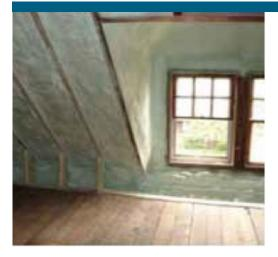
Attic room. This attic was insulated with spray foam at the roofline to provide additional conditioned living space in the home.
