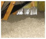
Loose fiberglass insulation
