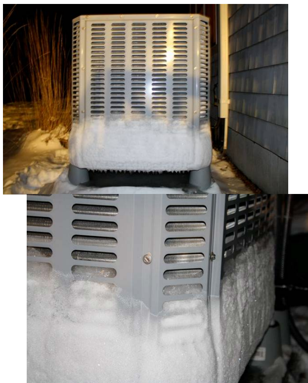
Figure 9. Ice accumulation on the outdoor coil. The ice was not removed during defrost cycles.
