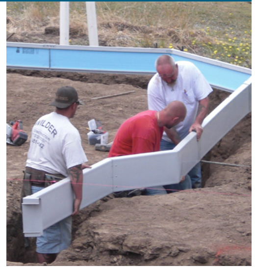
Davis Energy Group of the CARB Building America team developed a method for insulating slab perimeters. The method, which is commercially available, uses termicide-treated rigid foam insulation encased in PVC as the form for the concrete foundation.
