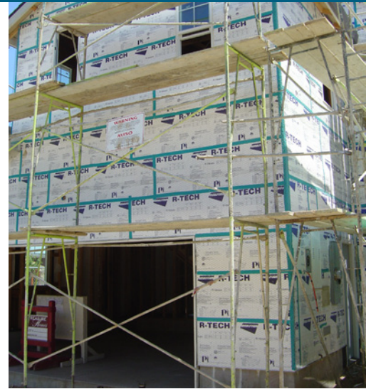
Treasure Homes of Sacramento installs rigid foam under stucco siding to serve as an insulation layer and exterior vapor barrier.
