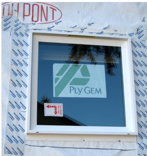
(top) Windows should be flashed in accordance with ASTM E2112-07.
