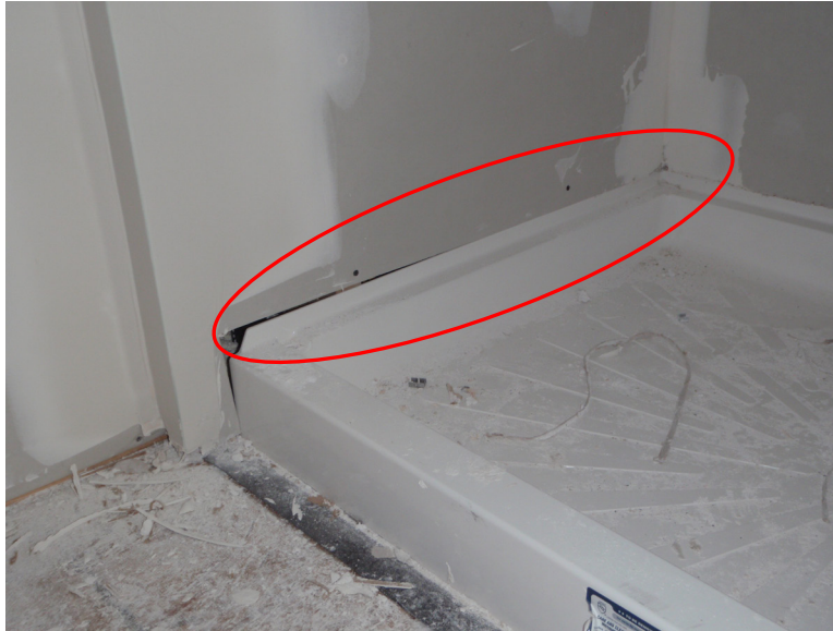
Figure 3. Acrylic shower pan with the backerboard installed above the nailing flange
