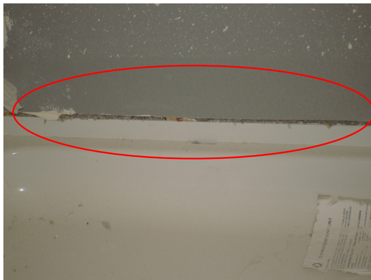
Figure 4. Gap between the backerboard and shower pan nailing flange that will be a direct water entry path into the wall assembly
