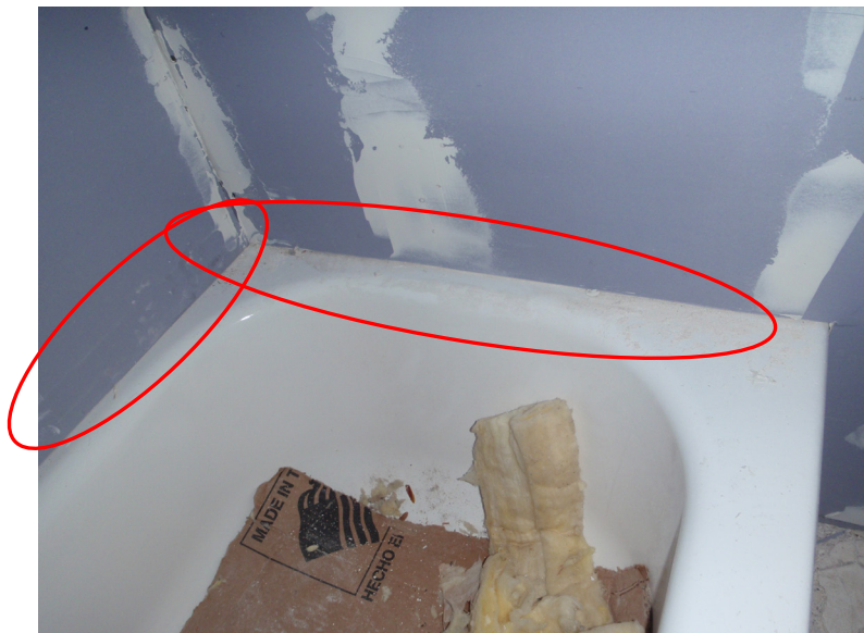
Figure 2. Backerboard material installed tight to the tub
