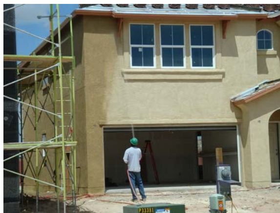
Figure 27. Hydration of the finish coat
