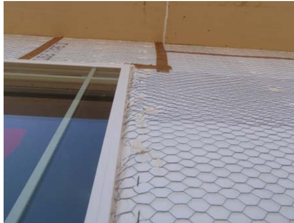
Figure 1. Beveling of EPS around a window
