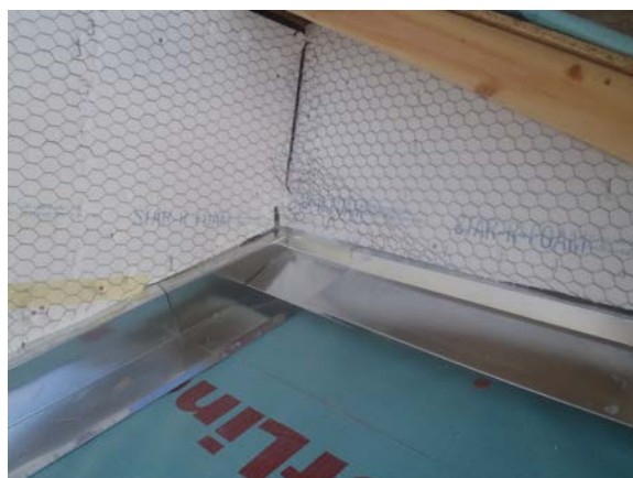
Figure 6. Flashing detail at roof-to-wall transition
