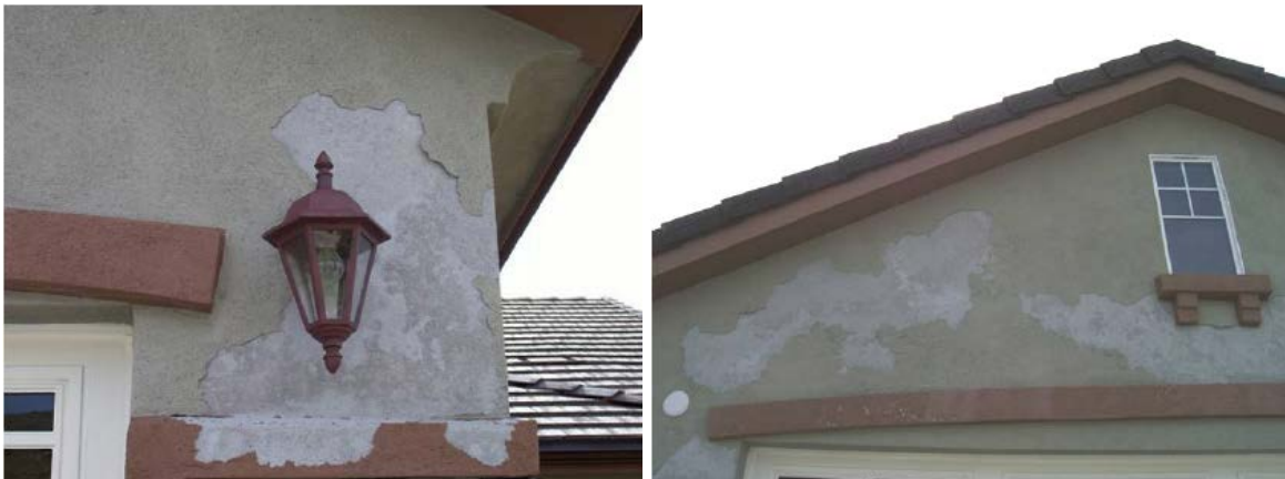
Figure 25. Delamination of stucco finish coat
