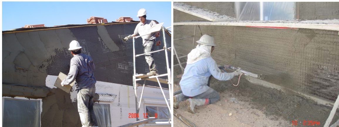
Figure 3. Application of stucco using trowels (left) and a stucco gun (right)
