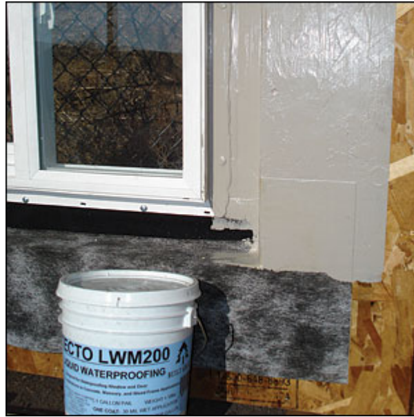
Figure 9. Liquid-applied coating as drainage plane and window flashing (Courtesy of Protecto Wrap)
