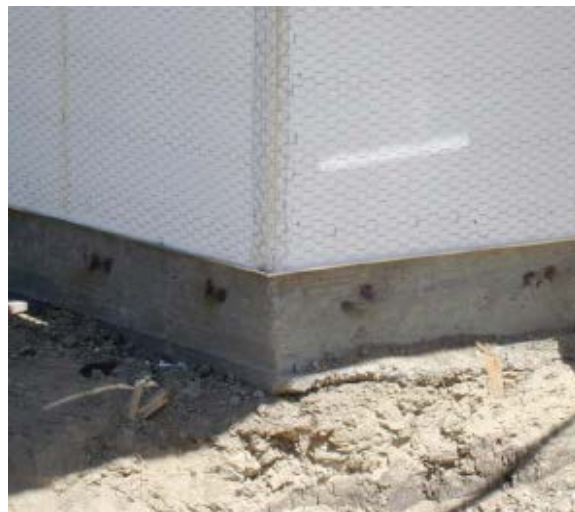
Figure 21. Properly installed corner bead (Courtesy of BuildIQ)
