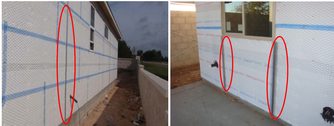
Figure 20. Expansion joints installed on a wall (left) and below a window (right)
