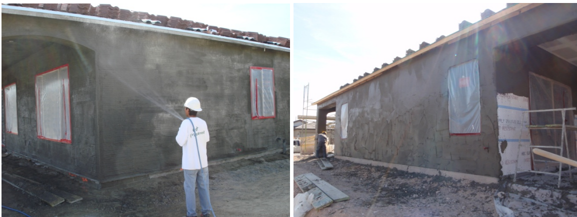
Figure 23. Hydrating (left) and curing (right) the stucco base coat
