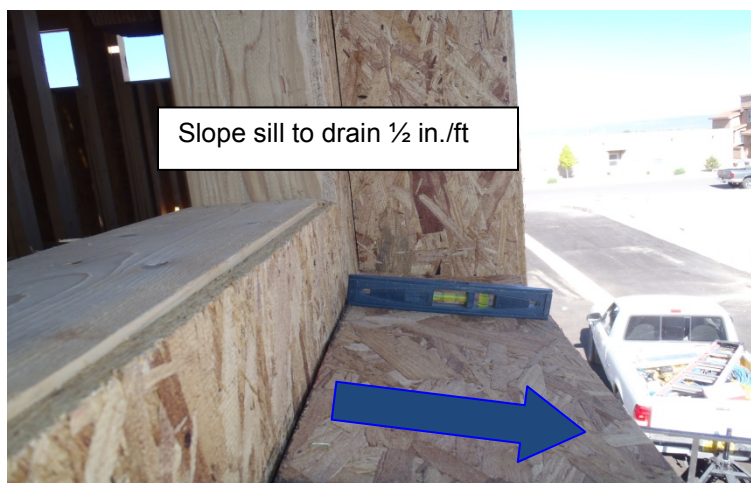
Figure 5. Proper sloping of recessed window sill
