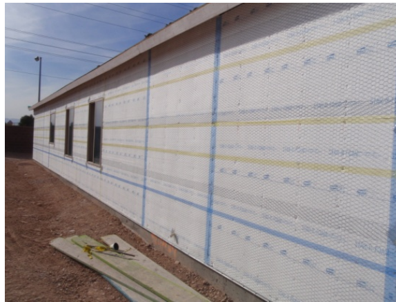
Figure 15. Proper installation of EPS bond break with taped joints
