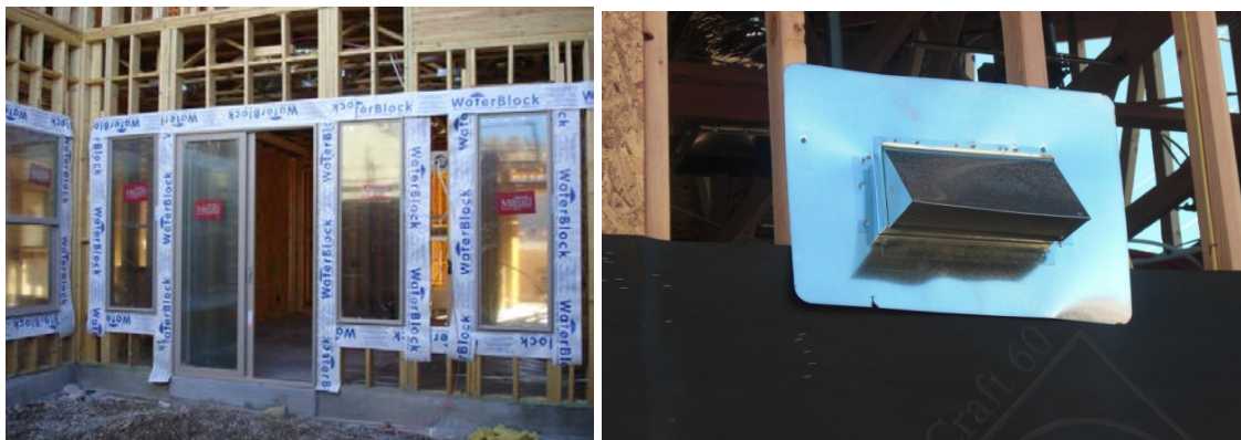
Figure 7. Proper flashing of window (left) and penetration (right) in a wall assembly
