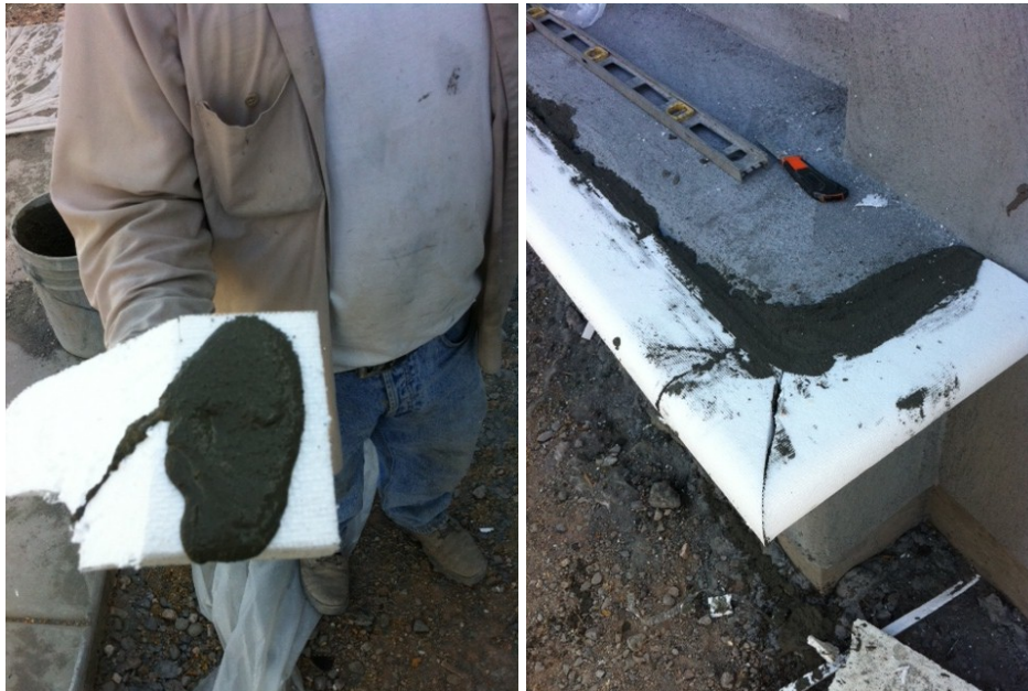
Figure 26. Architectural plant-on pieces being glued to a wall system
