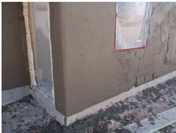
Figure 22. Stucco base coat during application
