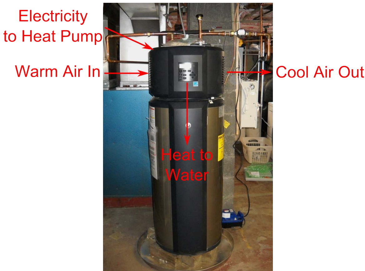
Figure 1. HPWH operation
