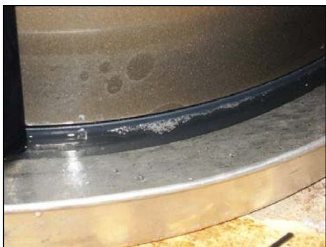
Figure 10. Condensate problems from improper installation
