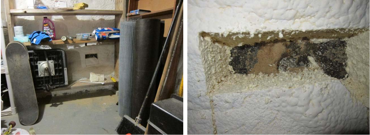
Figure 51. Test port cut into wall ccSPF, Bedford Farmhouse Renovation
