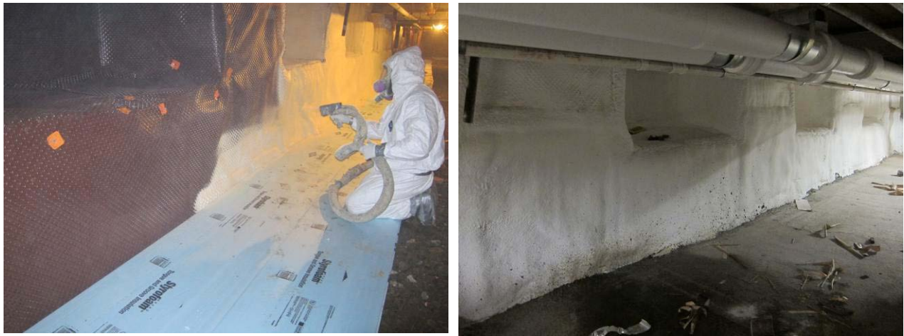
Figure 22. Spray foam slab edge insulation detail; completed installation of spray foam
