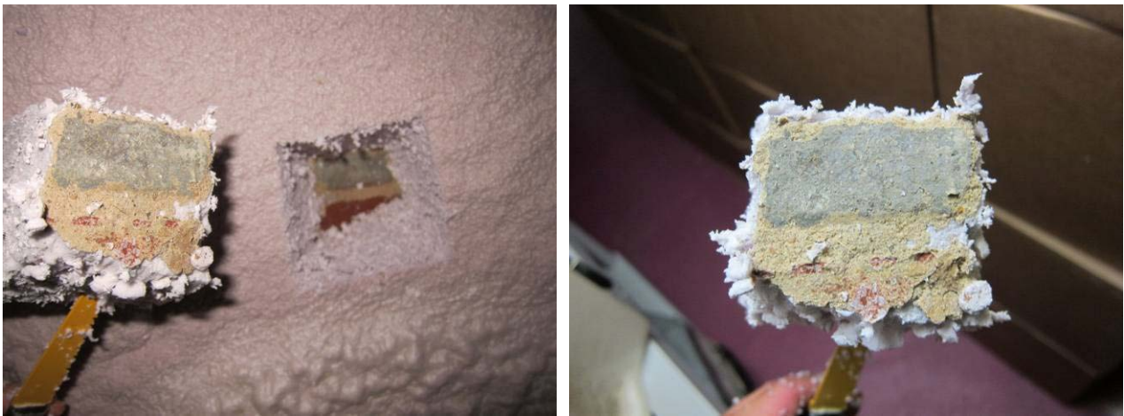
Figure 52. Test port cut into wall ccSPF, Somerville Office
