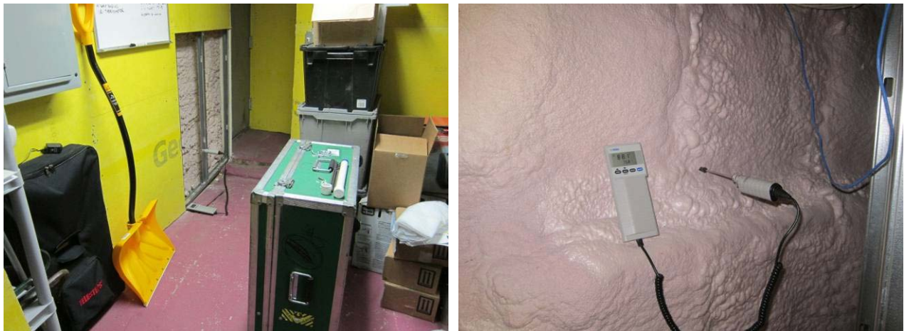
Figure 48. Measurement of T/RH conditions behind ccSPF insulation, Somerville Office
