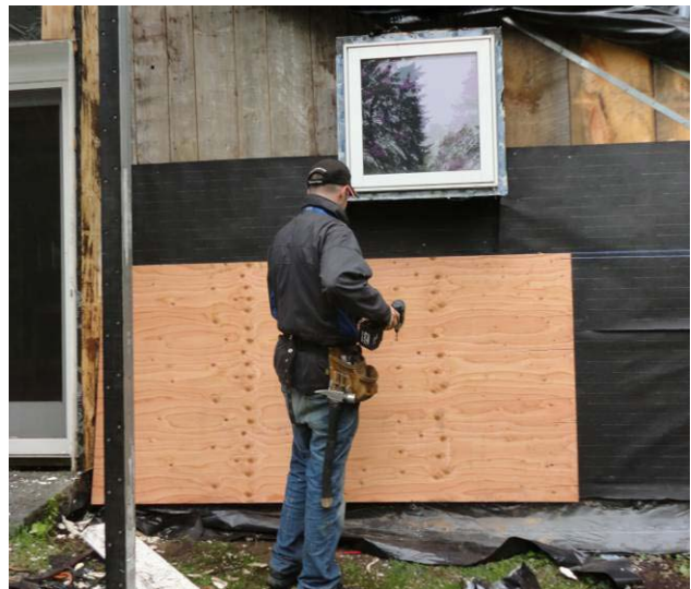
Figure 47. Westford House/Barn recladding and sill beam inspection
