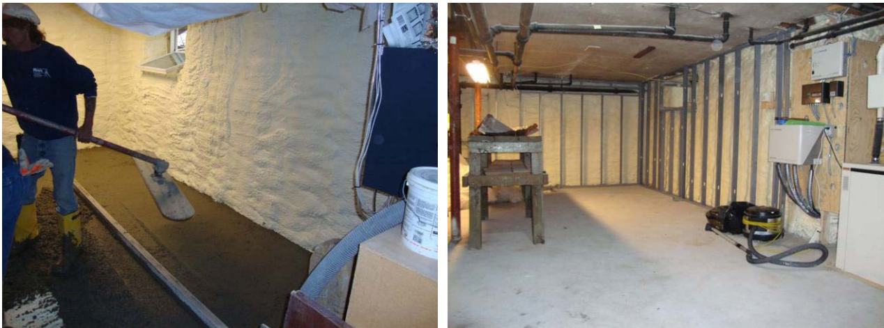
Figure 34. Casting of slab; wall framing (© 2011 by Byggmeister; reprinted with permission)
