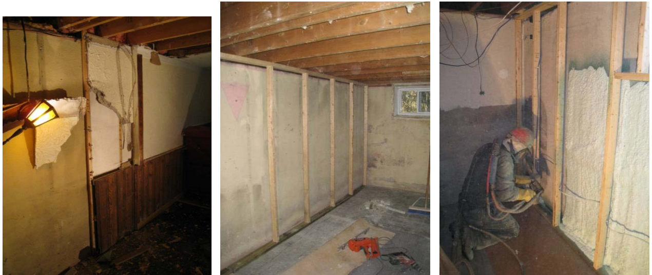
Figure 61. (L to R) Pre-retrofit basement; interior framing; spray foam application
