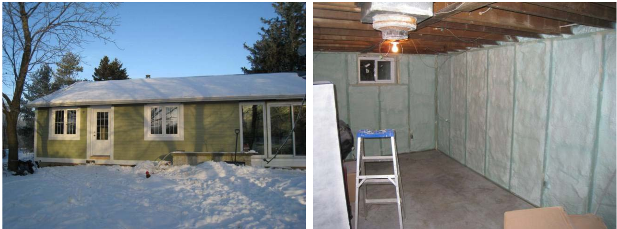
Figure 60. Exterior view of St. Agatha site; completed basement ccSPF retrofit
