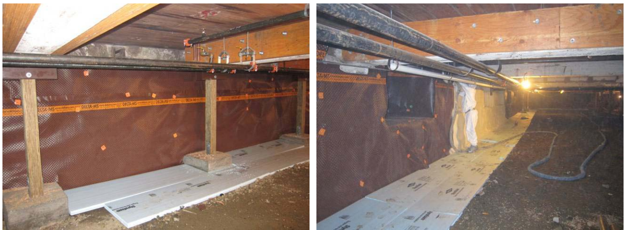
Figure 21. Air gap membrane under spray foam installation; 4’ basement slab edge insulation
