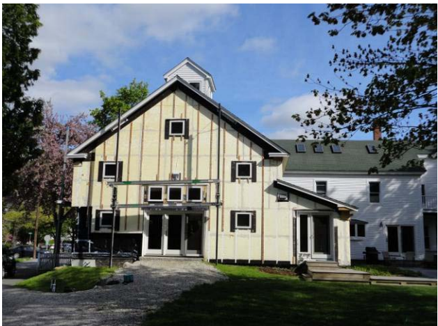
Figure 47. Westford House/Barn recladding and sill beam inspection
