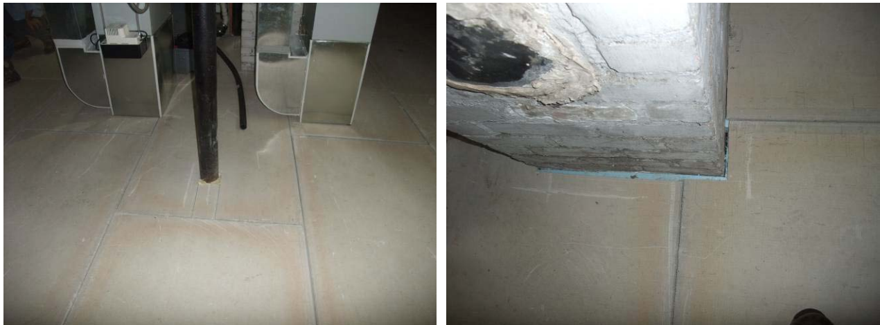
Figure 35. Storage use basement slab insulation/moisture control retrofit; cement board surface
