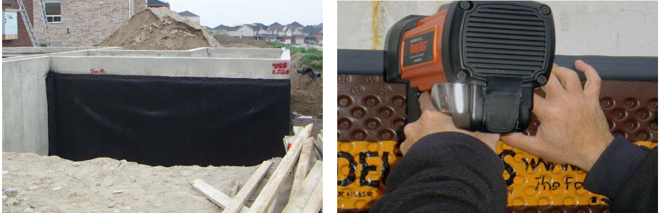
Figure 73. Air gap membrane below grade and top closure strip
