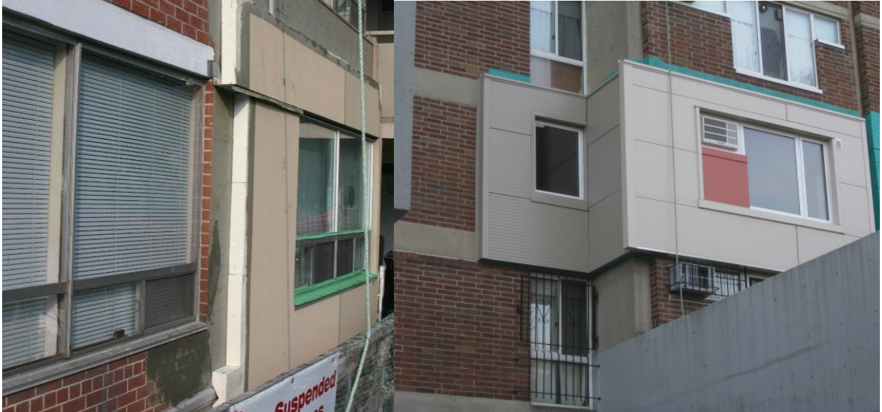
Figure 5. Exterior insulation retrofit approaches (Left: Exterior insulation and finish system; Right: Insulated metal panel cladding)
