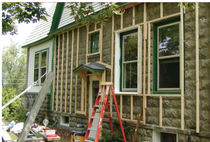
Figure 7. Exterior spray urethane foam retrofit on residential masonry
