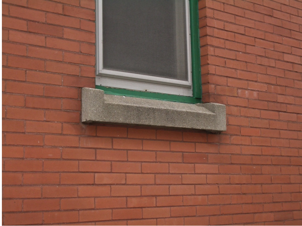
Figure 32. A high performance window sill, exhibiting end dams, steep slope, large projection, jamb extensions, and drip edge
