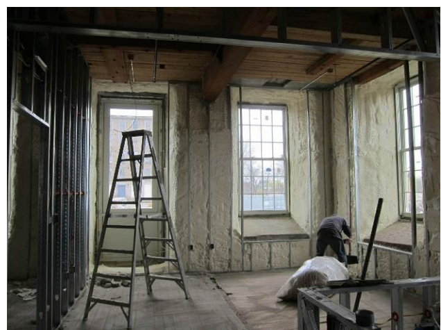
Figure 47. Window opening with tapered jamb detail (sill left uninsulated; not recommended)
