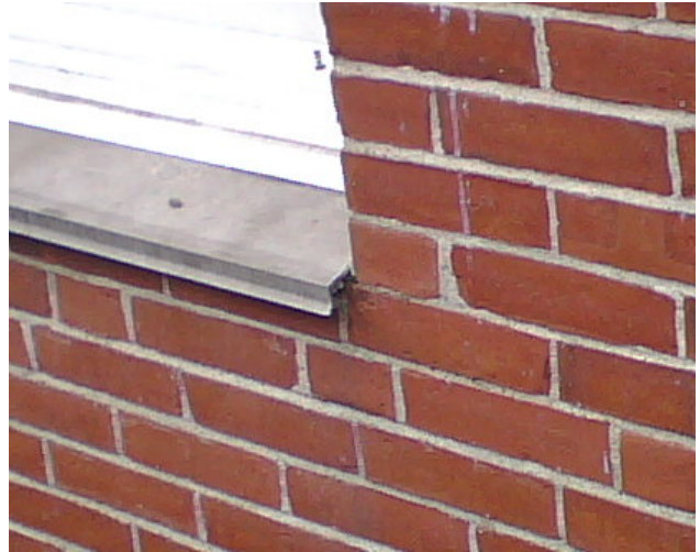
Figure 42. Example of overlaid sill detail (formed metal)
