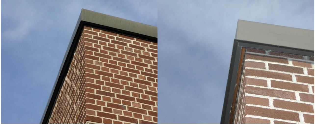
Figure 62. Improved drip edge overhang at coping
