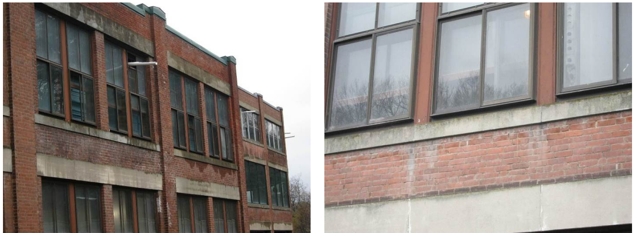
Figure 29. Improper drainage off window faces, and staining at window sill grout joints
