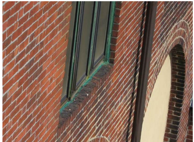
Figure 41. Left: Metal overclad detail of existing rowlock sill; Right: Original detail
