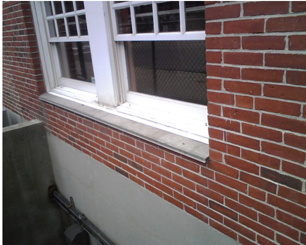
Figure 42. Example of overlaid sill detail (formed metal)
