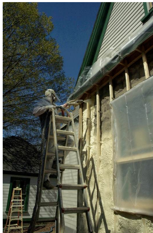
Figure 7. Exterior spray urethane foam retrofit on residential masonry
