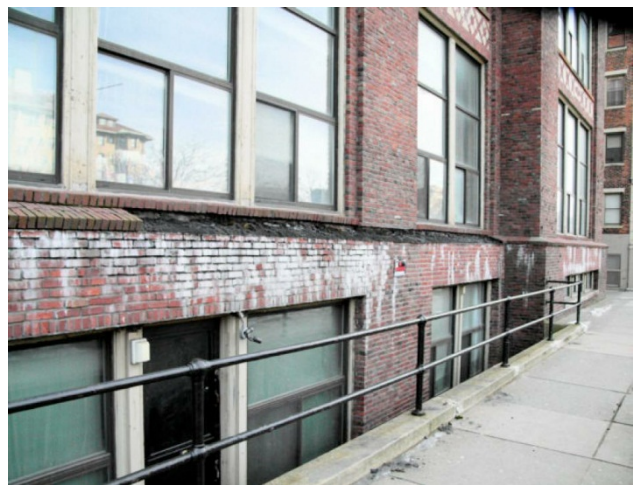
Figure 43. Left: Problem rowlock detail; Right: Failure of brick at detail
