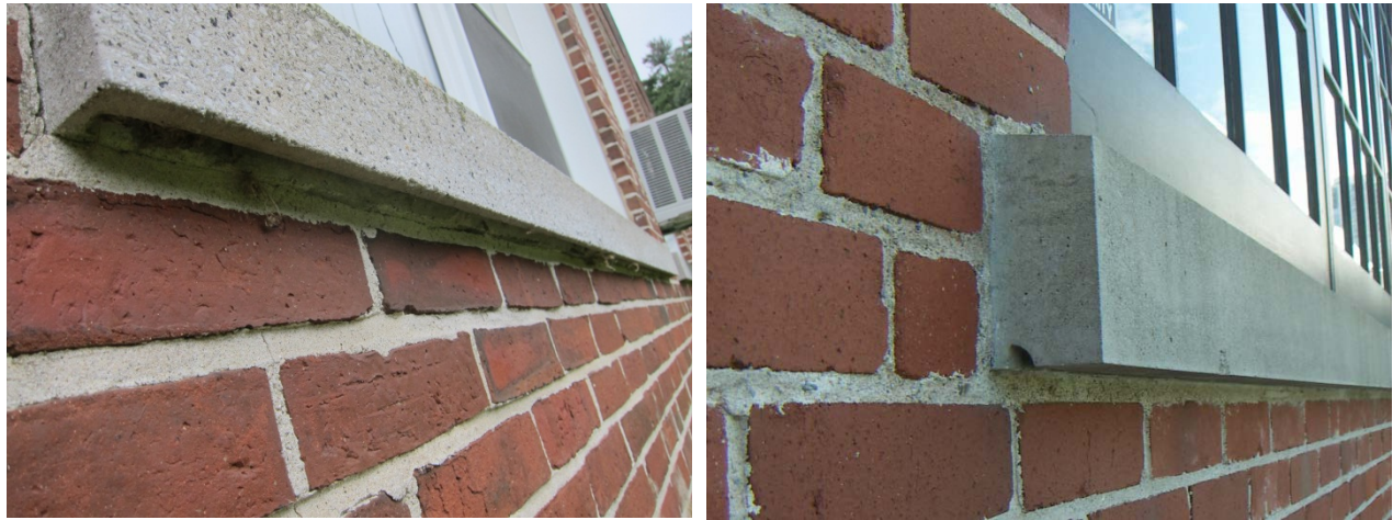
Figure 36. Precast window sill drip edge details
