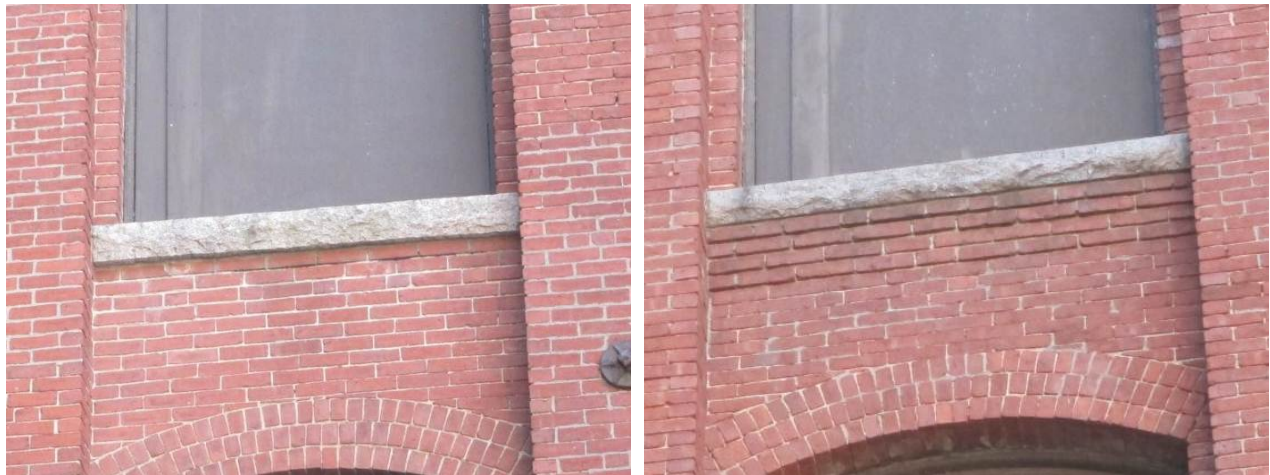
Figure 37. Left: Window sill without brick corbeling (left); Right: Window sill with brick corbeling, showing different mortar erosion patterns
