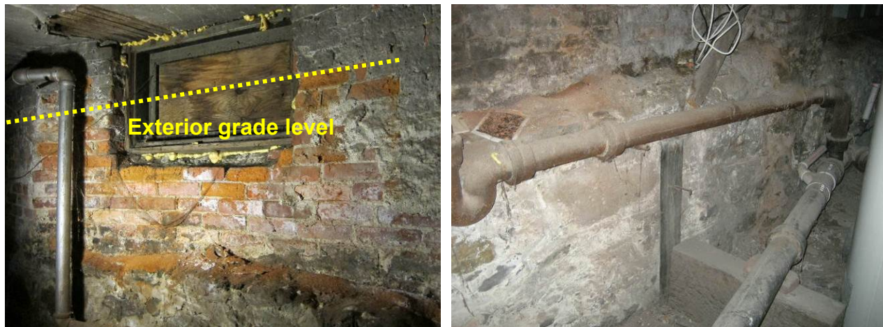
Figure 69. Left: Severe subfluorescence and spalling at basement window; Right: Stone shelf below grade
