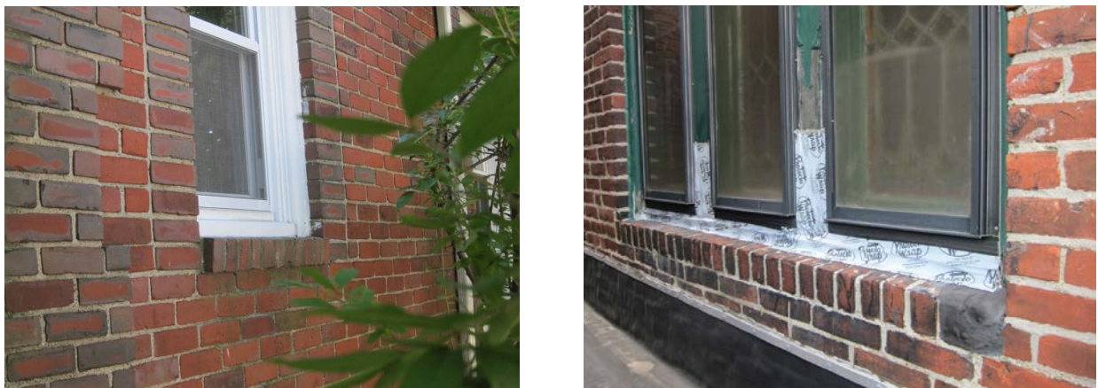
Figure 39. Rowlock window sill examples
