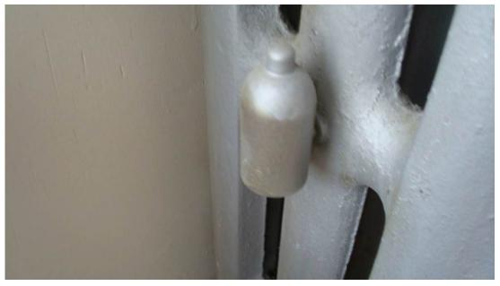
Figure 12. Painting over radiator vents is a common oversight that can have a serious effect on the heating in an apartment. Blocked radiator vents must be cleaned or replaced.
