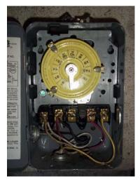
Figure 9. Time clock control for a steam boiler (used with permission from CNT Energy 2011)
