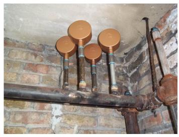
Figure 5. Main line air vents installed on a steam line. (used with permission from CNT Energy 2011)
