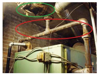
Figure 6. The header piping is smaller than the boiler manufacturer's specifications. (used with permission from CNT Energy 2011)
