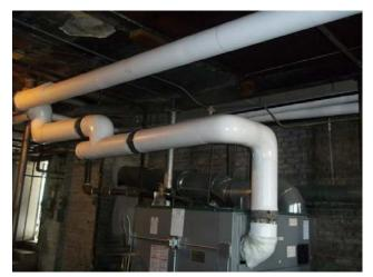
**Figure 8. Insulated heating pipes** (used with permission from CNT Energy 2011)
