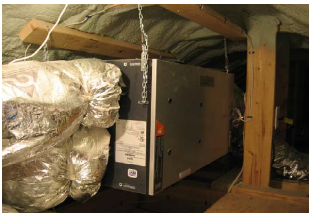
Figure 19. An HRV installed in a cold-climate home
