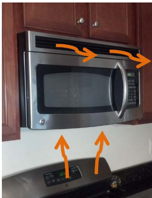
Figure 5. Some range hoods, like this one, do not vent outdoors. They simply circulate air back into the kitchen. Such hoods do not meet most ventilation requirements.
