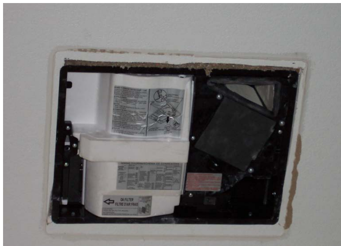
Figure 21. Local ERV (cover removed) installed in a home.
