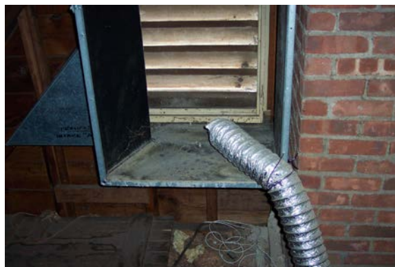
Figure 3. Exhaust ducts should always terminate outdoors—not in an attic “near” the outdoors.
