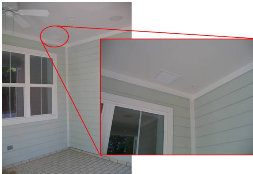
Figure 13. Poor location selection for CFIS ventilation intake, as the homeowners placed their outdoor grill in this corner of the patio
