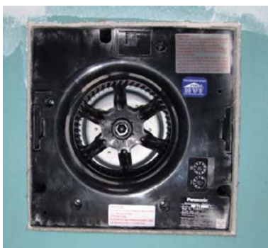
Figure 9. Many fans have adjustable speed settings (30–70 CFM in this fan) for continuous operation. When the bathroom is in use and more flow is desired, the fan can boost to 80 CFM for a preset time.
