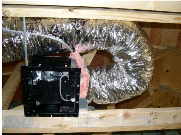
Figure 4. Tight bends can reduce fan flow rates, increase noise, and increase power consumption.
