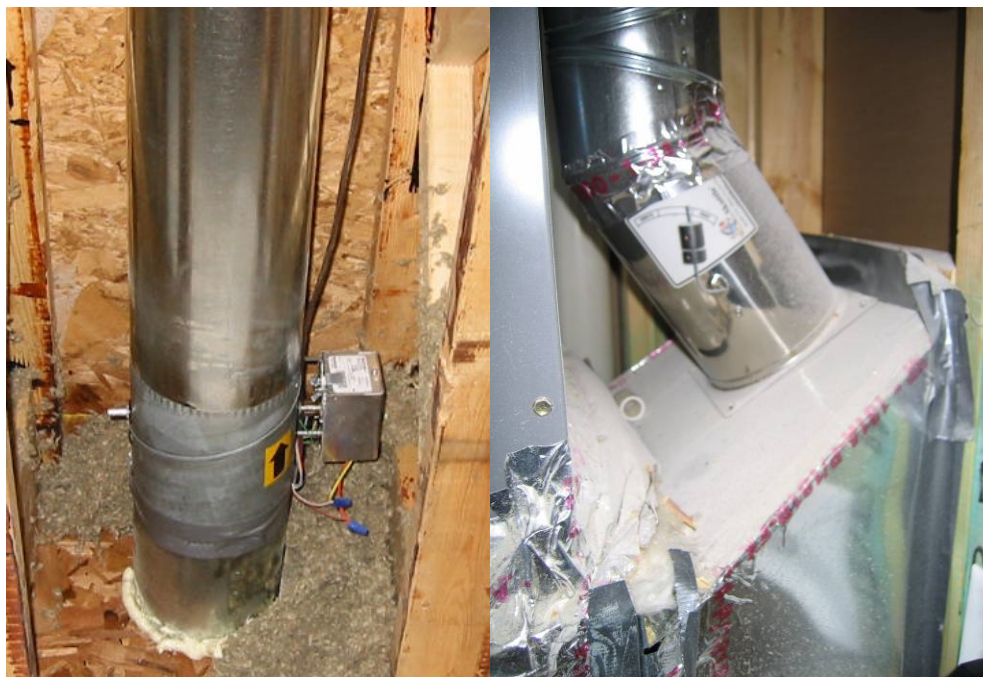
Figure 15. A motorized damper (left) and manual balancing damper (right) in CFIS systems
