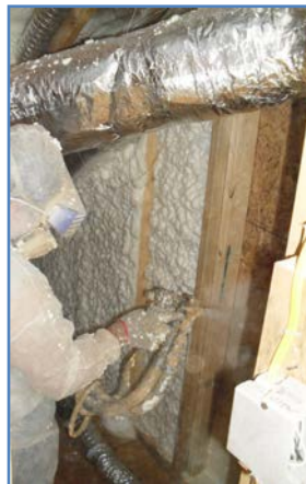
2. Apply foam to desired thickness following manufacturer's instructions
