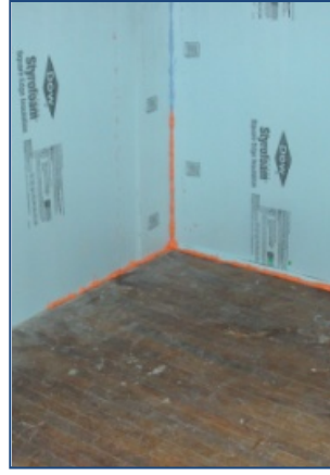
2. Install rigid foam and air seal.
