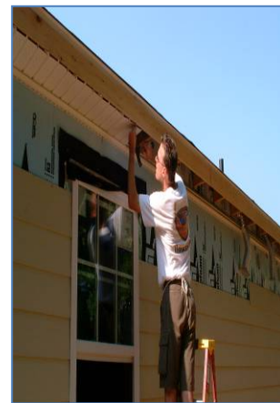
6. Install siding according to manufacturer's instructions.
