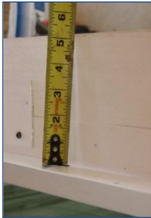
1. Extend door and window jambs as necessary.
