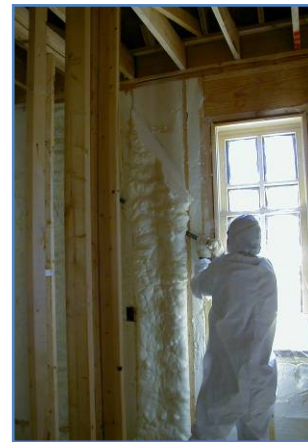
3. Remove excess foam if necessary
