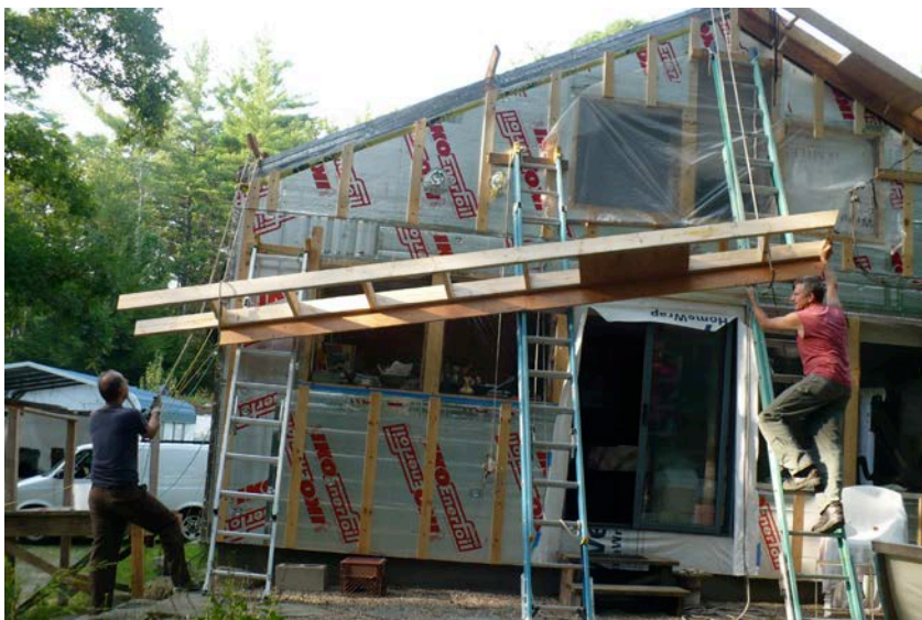
Figure 9. Pre-assembled insulated roof overhang framing being lifted into place at a gable rake for a “chainsaw” retrofit
