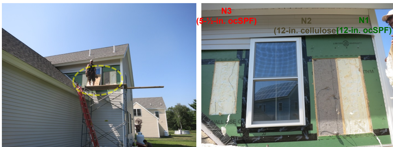
Figure 42. North-facing wall disassembly, showing test bay cavities
