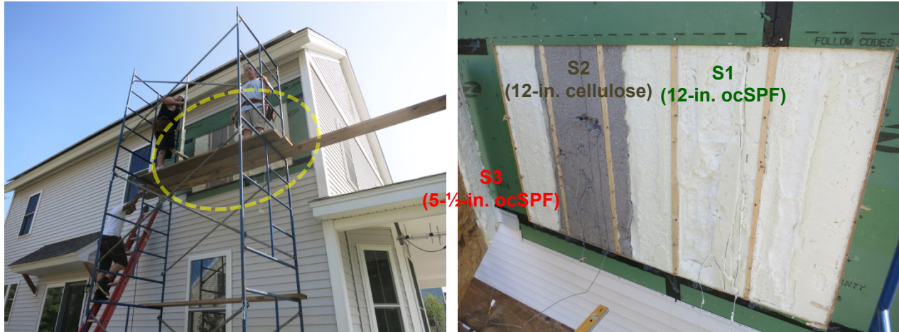
Figure 39. South-facing wall disassembly, showing test bay cavities
