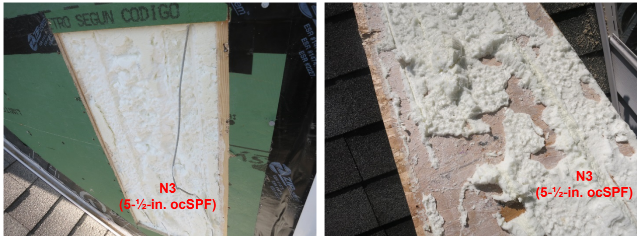
Figure 45. Stud bay cavity and sheathing conditions at 5-1/2-in. ocSPF north-facing wall (N3)
