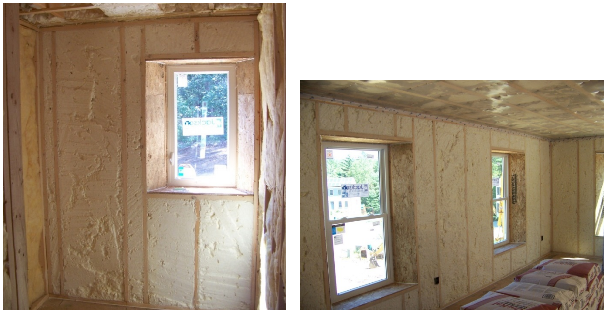
Figure 2. Typical installation of 0.5 lb/ft 3 (PCF) ocSPF in double-stud walls
