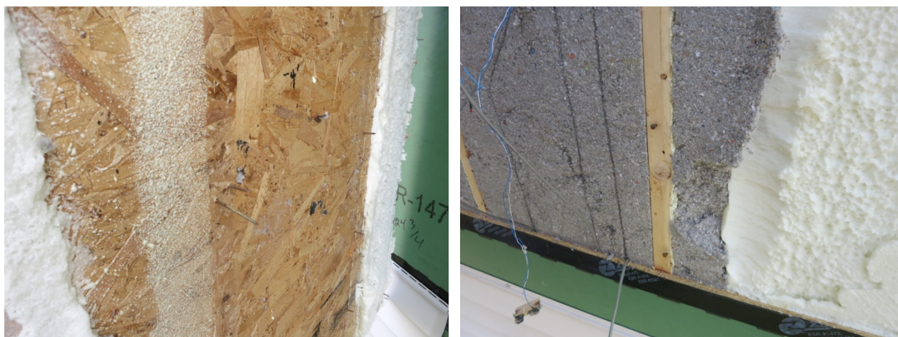
Figure 41. Sheathing and framing conditions at south-facing walls
