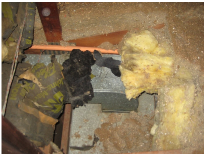
Figure 9. Supply trunk for third-floor apartment exposed to attic (pre-retrofit condition)
