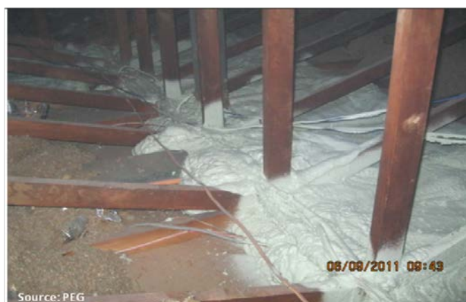
Figure 9. Membrane application followed by SPF application to seal off top of duct bulkhead from attic
