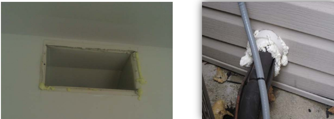
Figure 6. Air sealing of duct register boot and an HVAC penetration
