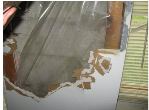
Figure 3. Polyethylene layer on inside face of concrete masonry unit (CMU) wall assembly
