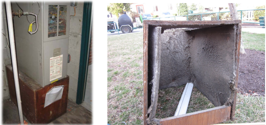
Figure 8. Pre-retrofit HVAC return plenum
