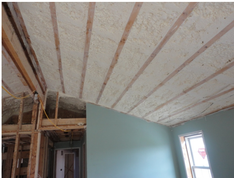
Figure 2. Spray foam insulation used for air control in rafter cavities (with cross strapping)
