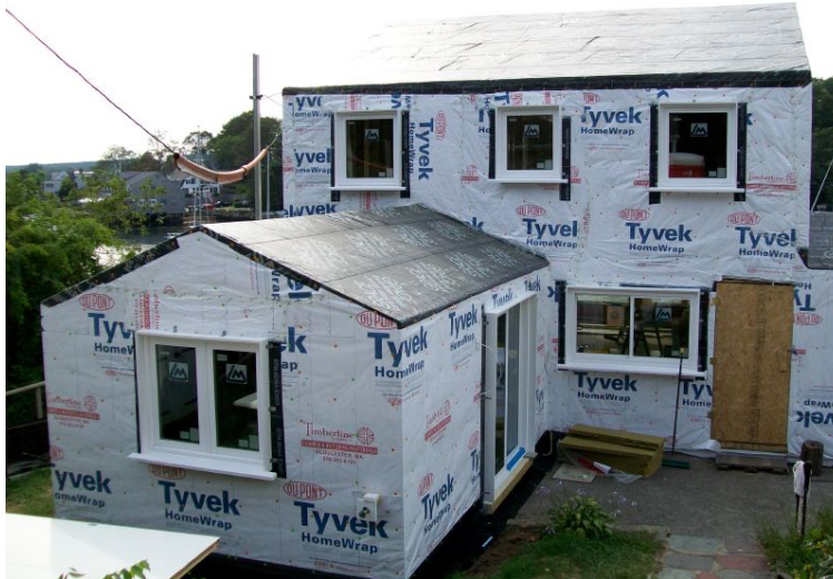
Figure 1. Chainsaw retrofit with fully adhered roofing membrane and house wrap as the air control layers
