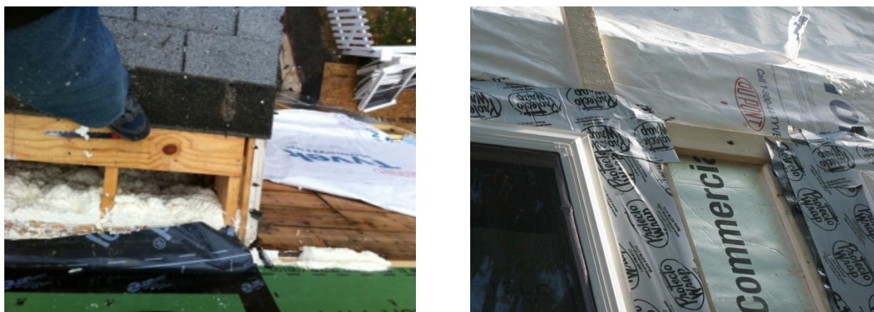
Figure 13. Left: Attached roof cut back to allow application of ccSPF at roof-wall interface; Right: Window flashing problems associated with installation of windows over strapping.
