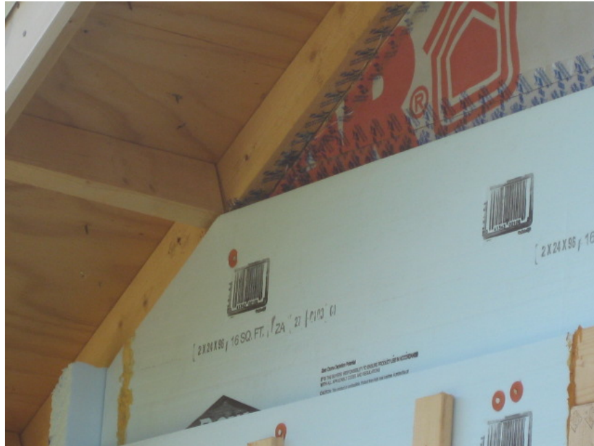
Figure 32. Example of airflow control transition at gable end of vented attic. The house wrap is taped to the wall sheathing at the level of the attic floor. Note that it is not necessary to tape the house wrap above this level.
