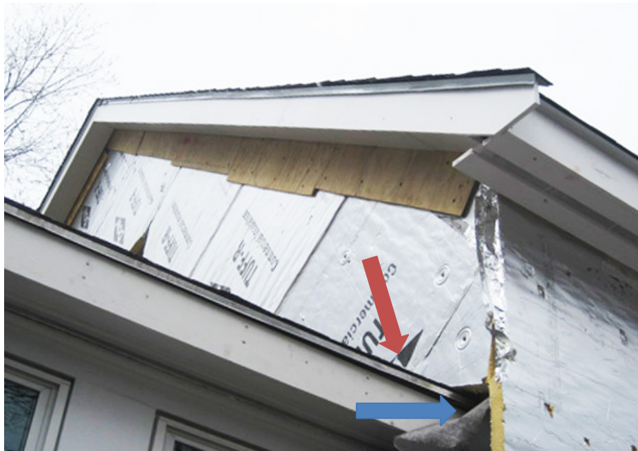
Figure 35. Wall-roof interface at Test Home 4 showing two common flashing errors: 1) step flashing is not located at plane of water control, and 2) drip edge of lower roof creates a condition where water may be directed in behind the drainage plane. Note that both of these conditions were corrected at this test home.
