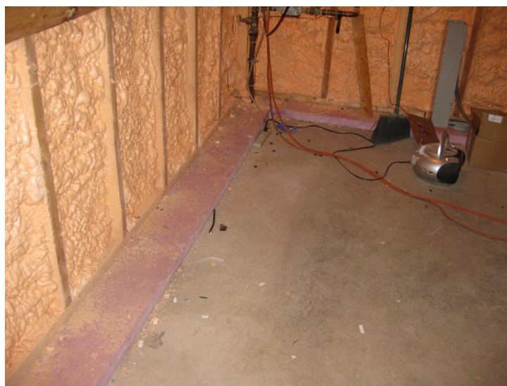
Figure 54. Thermal break between wood stud wall and existing concrete slab at Test Home 1
