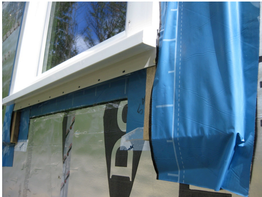
Figure 50. Installation of the window over strapping provides a generous drainage gap for the sill pan flashing.
