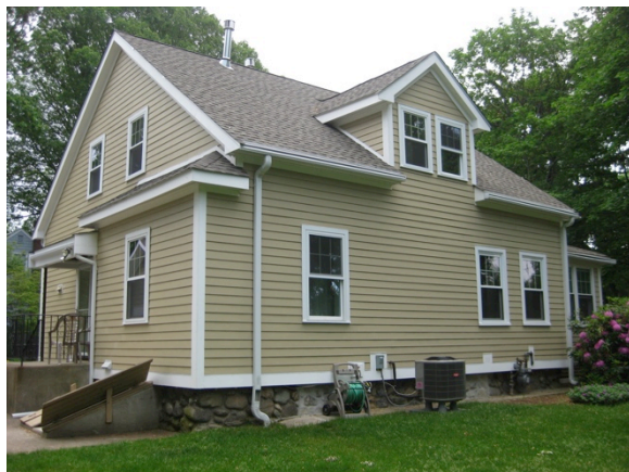
Figure 27: Left and Right: Test Home 4 after implementation of the DER project. Note the generous main roof overhangs and the overhangs of the dormer roofs that are slightly larger than they had been prior to the DER.
