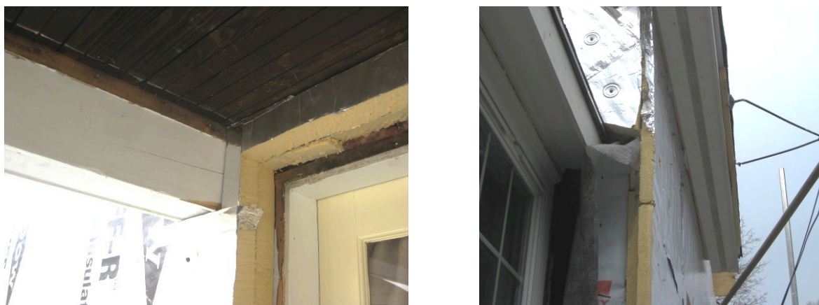
Figure 39. Left: Porch roof support beam with trim and porch ceiling void airflow control where they connect to the wall and penetrate exterior insulation; Right: A porch roof return that connects to the existing wall challenges continuity of airflow control.
