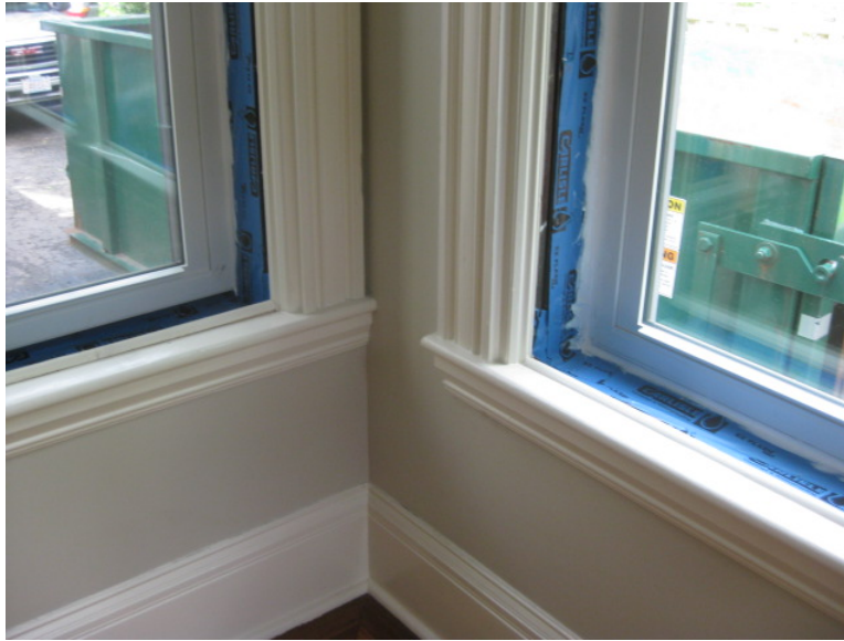
Figure 52. Window sealed to membrane at inside perimeter of window at Test Home 2. Note how the window frame is slightly larger than the finished opening.
