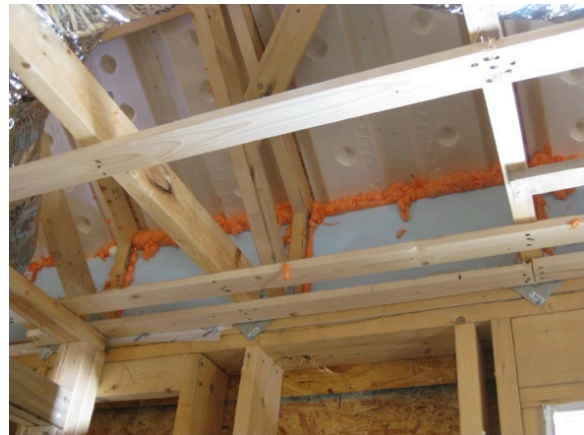
Figure 34: Left: Rigid insulation blocking between roof trusses at Test Home 5 exterior; Right: Rigid insulation blocking between roof trusses at Test Home 5 interior
