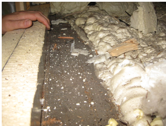
Figure 47. Left: Top plate at insulated ceiling showing new rigid insulation to other side of top plate, Test Home 2; Right: Top plate between previously retrofit ceiling and newly retrofit wall, Test Home 2
