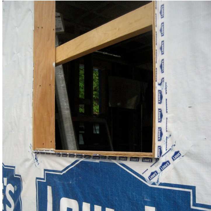
Figure 43. House wrap airflow control layer sealed to window extension box at Test Home 5
