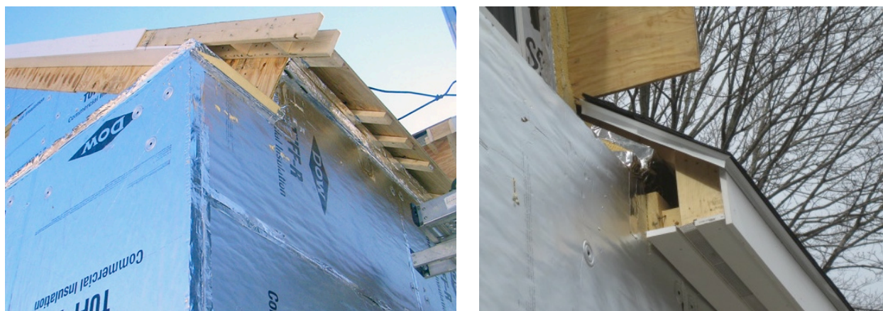
Figure 28. Left: Plywood gable rake support at Test Home 4. Right: fascia and soffit of main roof framed over insulation layers and attached to 2 × 4 purlins.
