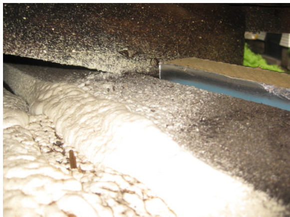
Figure 47. Left: Top plate at insulated ceiling showing new rigid insulation to other side of top plate, Test Home 2; Right: Top plate between previously retrofit ceiling and newly retrofit wall, Test Home 2
