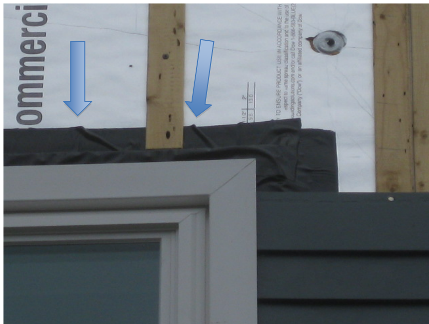
Figure 49. Wrinkles in flashing membrane wrapped over strapping and back to drainage plane. Note how this window head flashing requires flashing of its own.
