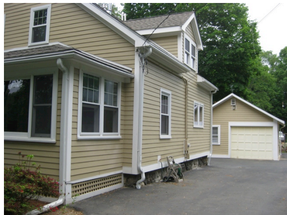
Figure 27: Left and Right: Test Home 4 after implementation of the DER project. Note the generous main roof overhangs and the overhangs of the dormer roofs that are slightly larger than they had been prior to the DER.
