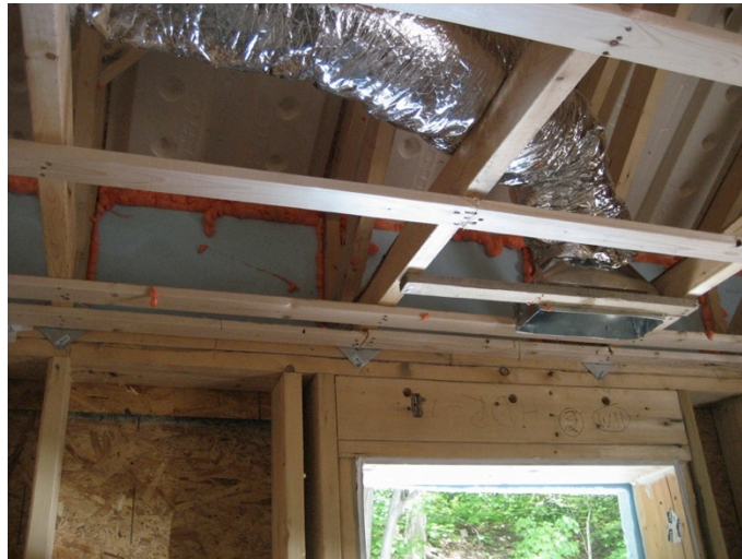
Figure 30. Ventilation duct initially located above airflow control layer in vented attic at Test Home 5
