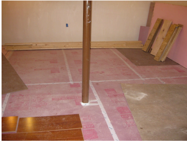
Figure 56. Basement floor insulation at Test Home 1 installed near end of project to prevent damage to insulation
