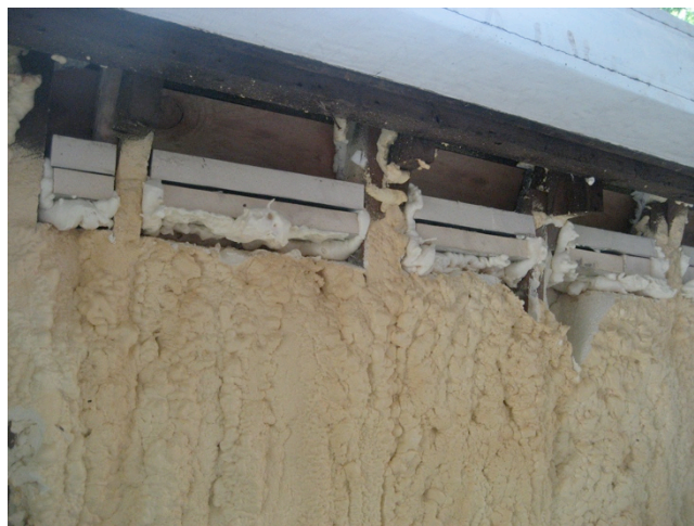
Figure 46. Left: Front of building showing overhang during retrofit work, Test Home 2; Right: connection between new work and previous work at wall-overhang interface, Test Home 2
