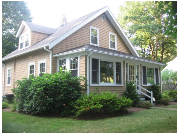
Figure 26. Left and Right: Test Home 4 prior to implementation of the DER project. Note the generous main roof overhangs and the smaller overhangs of the dormer roofs.
