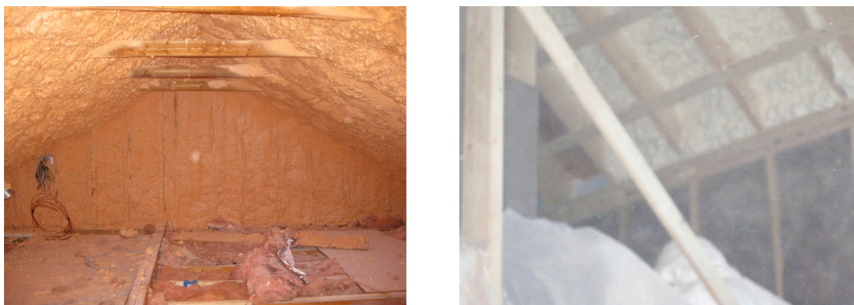
Figure 19. Left: ccSPF insulated roof at Test Home 1; Right: partial ccSPF insulation in a section of roof framing at Test Home 3. Note that Test Home 1 remained unoccupied except for active construction for a period of several months after application of ccSPF. During active construction, doors and windows remained open. During the period after application of ccSPF in Test Home 3, the application floor and floor below were active construction zones with doors and windows typically open during daytime hours.
