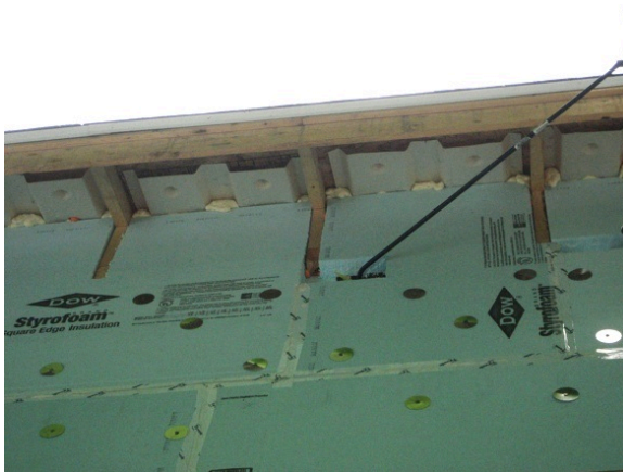
Figure 34: Left: Rigid insulation blocking between roof trusses at Test Home 5 exterior; Right: Rigid insulation blocking between roof trusses at Test Home 5 interior
