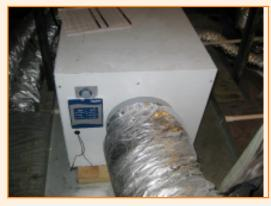
dehumidification through standard cooling during periods of high cooling. Initially, the 90 pint Aprilaire® Model 1750 dehumidifier's operation dial was set in the 3-5 range, per the manufacturer's installation manual. This was too high of a setting and it resulted in the dehumidifier running too much. The 90 pint unit outputs around ~10 kBtu while operating. This was
