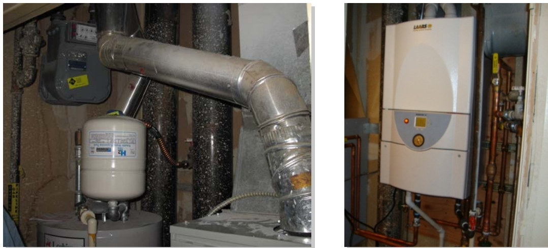
Figure 4. Space and water heating systems pre- and post-retrofit
