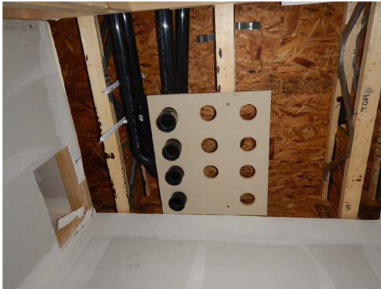
Figure 30. Ceiling support guide
