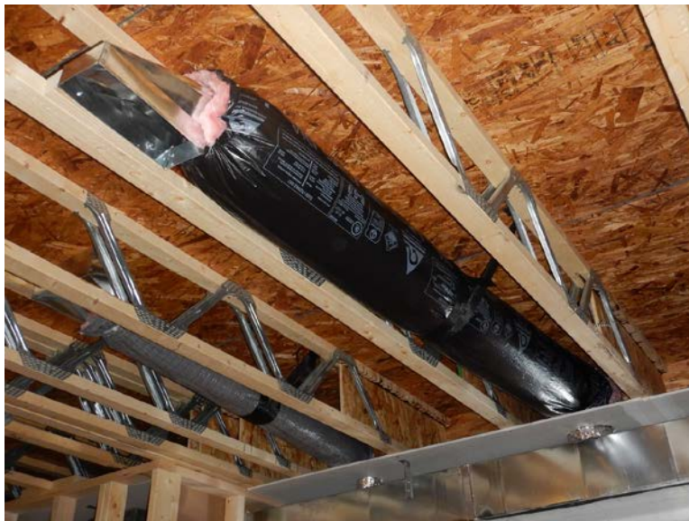
Figure 19. Six-inch branch duct
