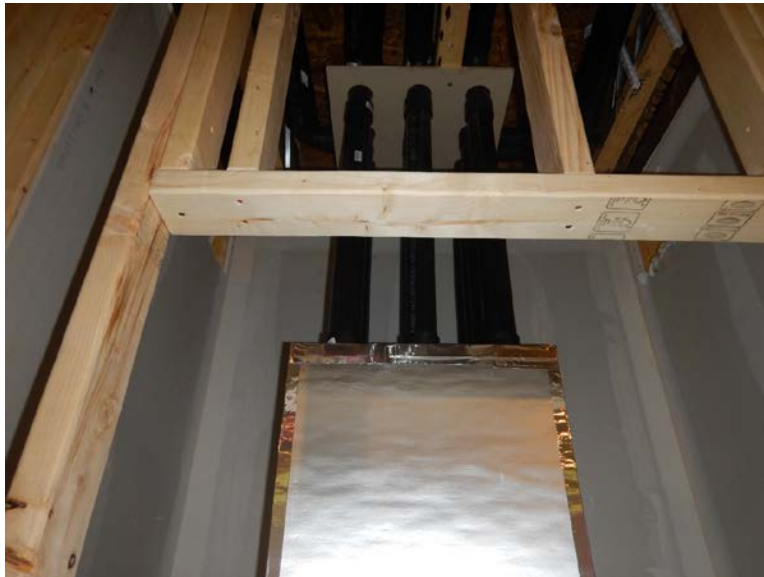
Figure 32. Final connections at the manifold
