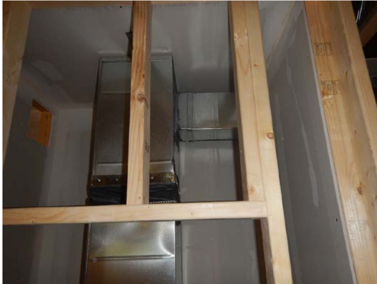
Figure 18. Riser plenum and side takeoff
