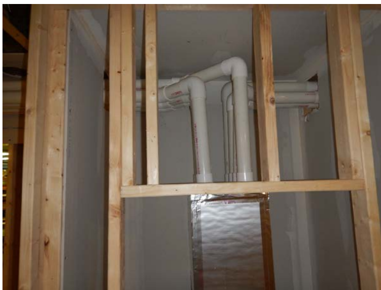
Figure 27. Final connections at plenum manifold
