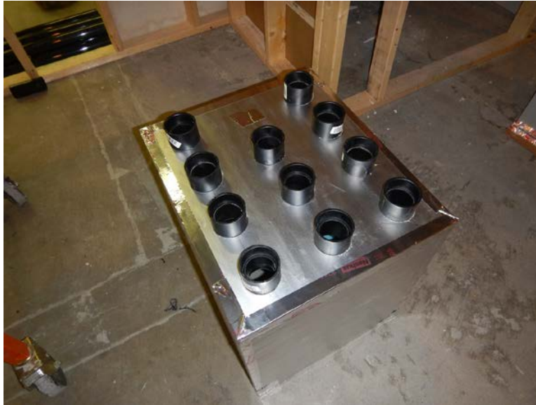
Figure 31. Two-inch PnP manifold
