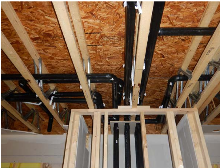
Figure 33. Pipe distribution through floor
