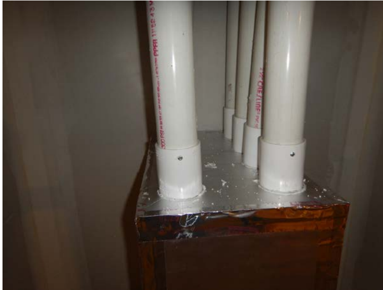
Figure 24. Plenum manifold with takeoffs
