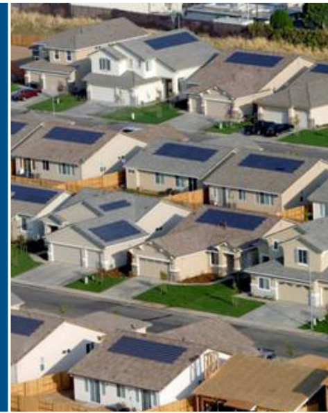
A view of the 95 homes of Premier Gardens, all today's zero energy. Photo courtesy of Sacramento Municipal Utility District.
