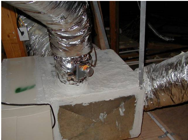
Figure 28. 6 in. Normally Closed 24V motorized damper installed
