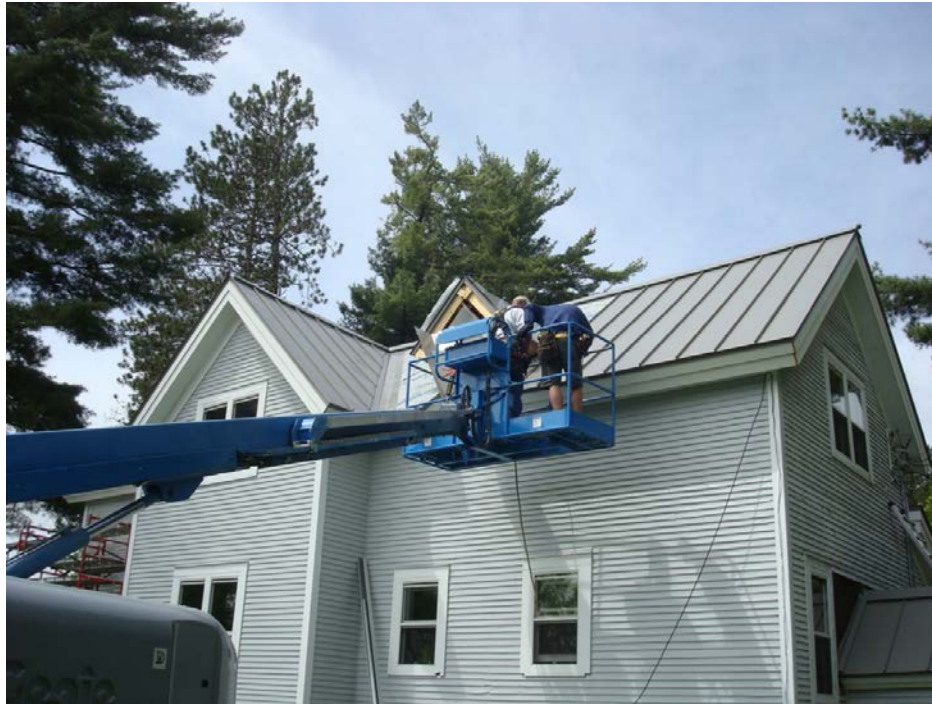
Figure 29. SIP retrofit panel installation with double fascia
