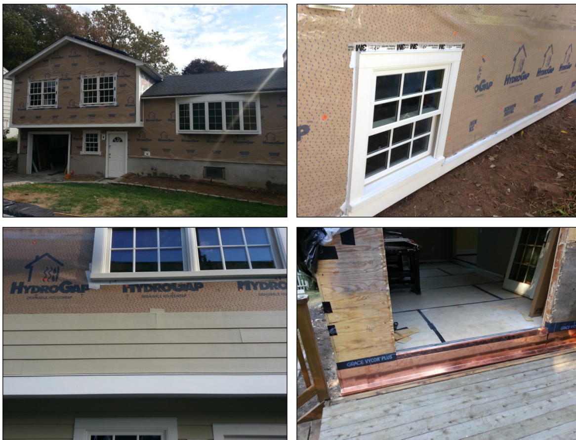
Figure 9. Continuity of the drainage plane: a dimpled WRB was applied over the sheathing (upper left); windows were properly flashed and drip edges were installed over all windows, doors, and trim board (upper right); a door pan and flashing were used to prevent further water damage at the rear sliding door (lower right); fiber-cement siding was installed over the WRB (lower left).
