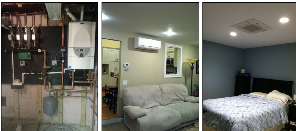
Figure 11. Mechanical equipment updates: new natural gas combi-boiler provides heat to the hydronic baseboards and for DHW (left); wall-mounted indoor unit for the multiport heat pump provides air conditioning for family room (center); ceiling cassette indoor unit provides air conditioning and auxiliary heating for bedroom (right).
