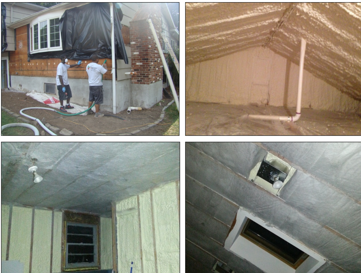
Figure 10. Continuity of the thermal barrier: dense-packed cellulose blown into the walls from the exterior (upper left); the vented attic over the bedrooms was being used as cold storage, so this space was converted to warm storage by applying ccSPF to the roof deck to make an unvented attic (upper right); the vaulted ceiling drywall was removed to allow for 3 in. of ccSPF to be applied to the roof deck before dense packing the remainder of the roof rafters with cellulose (lower right); drywall from the garage was removed to allow the bedroom floors to be properly insulated and to isolate the garage contaminants from the living space (lower left).
