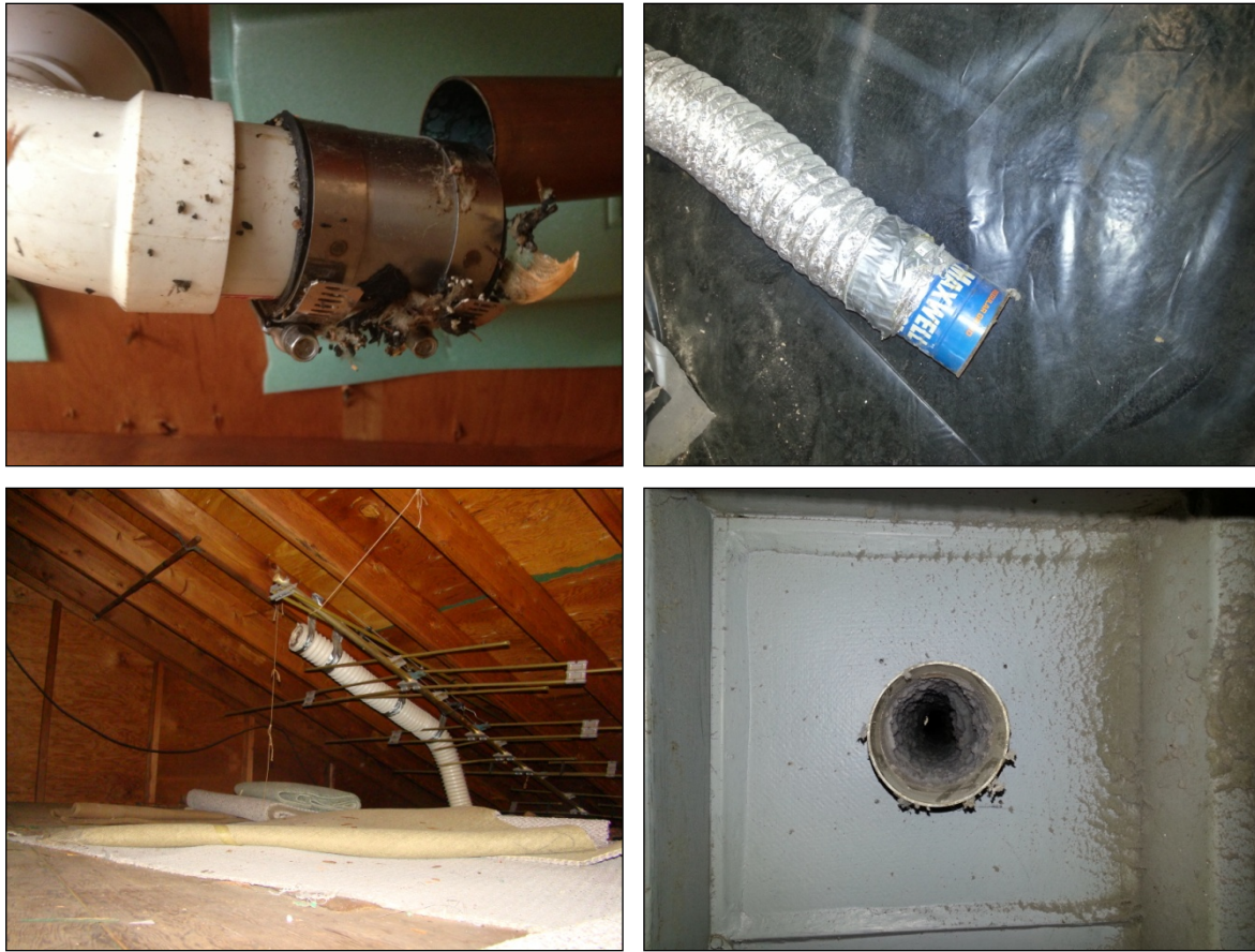
Figure 6. Piping/duct hazards: disconnected plumbing vent pipe (upper left); coffee can used as clothes dryer vent splice (upper right); clothes dryer exhaust duct was lined with a significant amount of lint (lower right); the second-floor bathroom exhaust terminates in the unvented attic (lower left).
