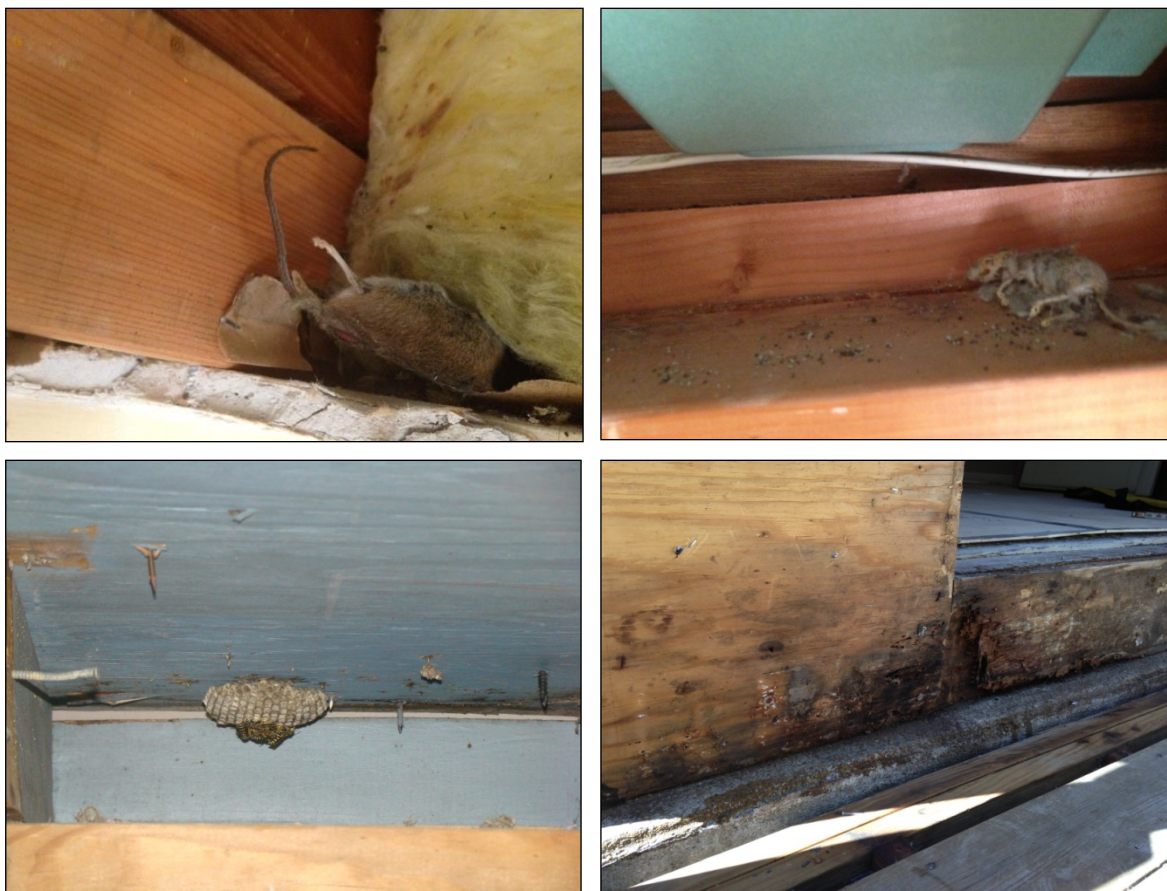
Figure 5. Pest hazards: dead mice were found in the vented attic space over the bedrooms and in the vaulted ceilings (upper right and left); active wasp nests were found throughout the soffit eaves and in several cases had a pathway into the home (lower left); termites had started to infest the exterior wood components under the rear French doors (lower right).
