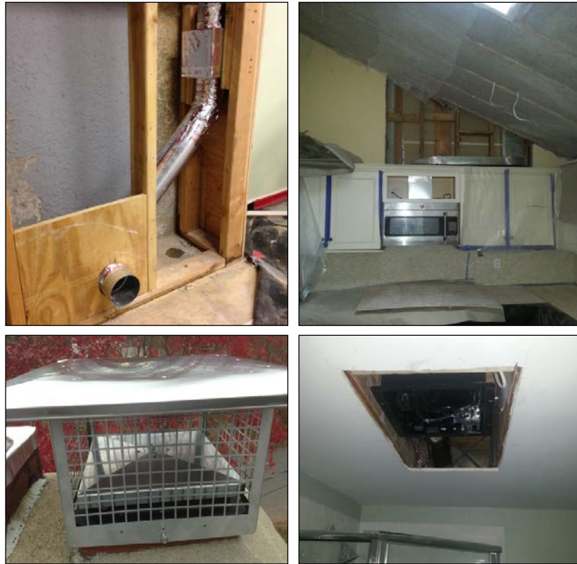
Figure 12. Additional improvements: a secondary lint trap was installed on the clothes dryer (upper left); the microwave over the kitchen range was exhausted to outdoors (upper right); an exhaust fan was added to the first-floor bathroom that had no fan or window previously (lower right); a lock-top chimney damper was installed on the wood-burning fireplace (lower left).
