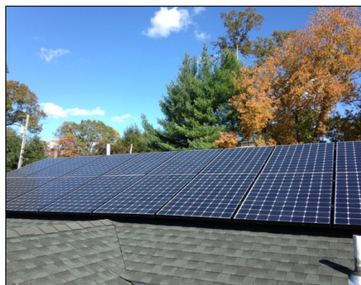
Figure 13. A 5.2-kW PV system was installed on this 1960s retrofit project.
