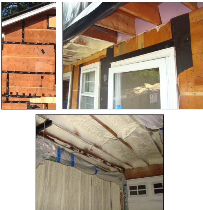
Figure 8. Air-sealing details: all seams and penetrations in exterior sheathing were taped (upper left); blocking was installed to eliminate cold air from the overhang from entering the floor system (upper right); the attached garage was isolated from the living space with ccSPF (lower center).
