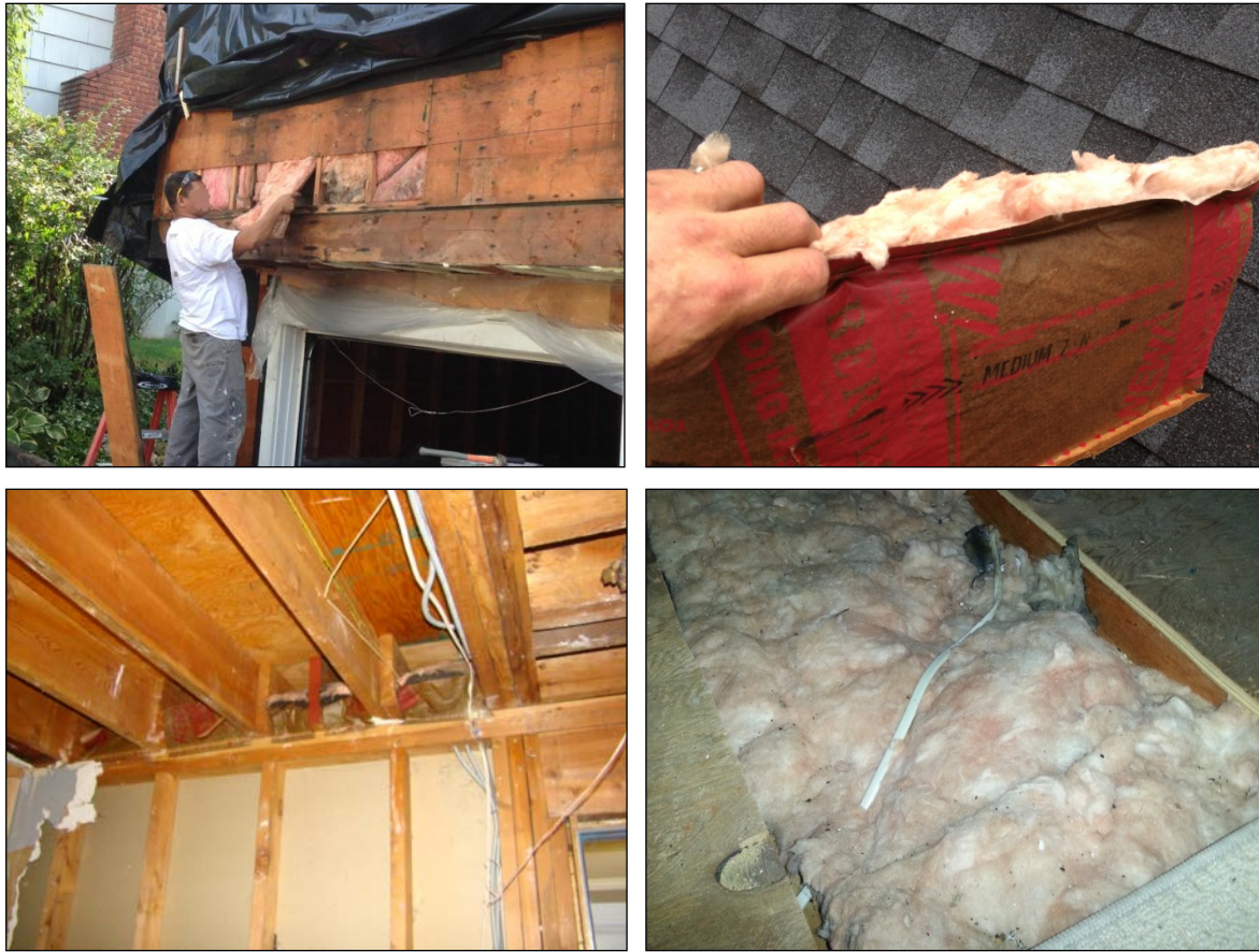
Figure 2. Pre-retrofit insulation conditions: exterior wall insulation being pulled from exterior (upper left); wall insulation thickness (upper right); attic insulation (dead rodents were a major issue during this retrofit) (lower right); garage ceiling insulation (no air blocking between conditioned parts of home) (lower left).
