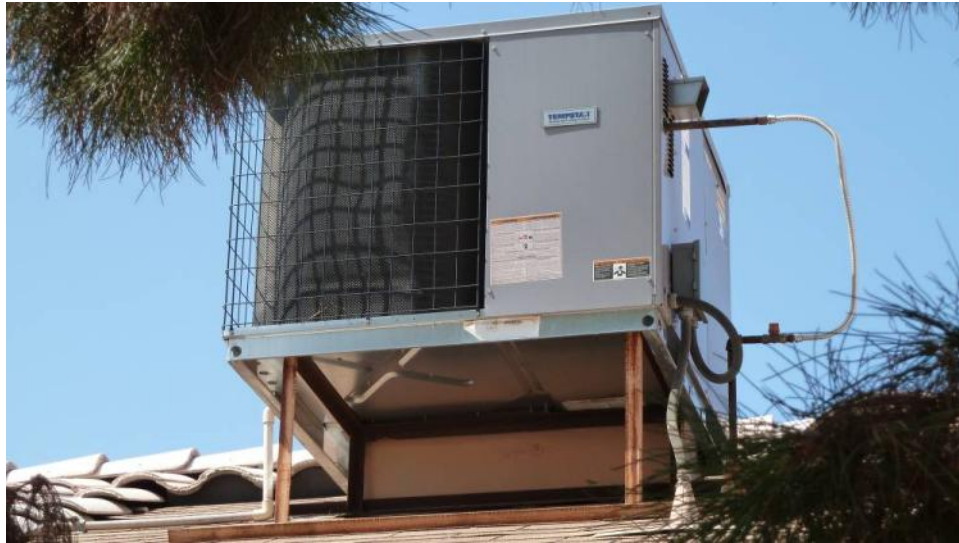
Figure 15. Rooftop packaged furnace/AC located at the Sierra Hills home (Image courtesy of Building Media, Inc.)
