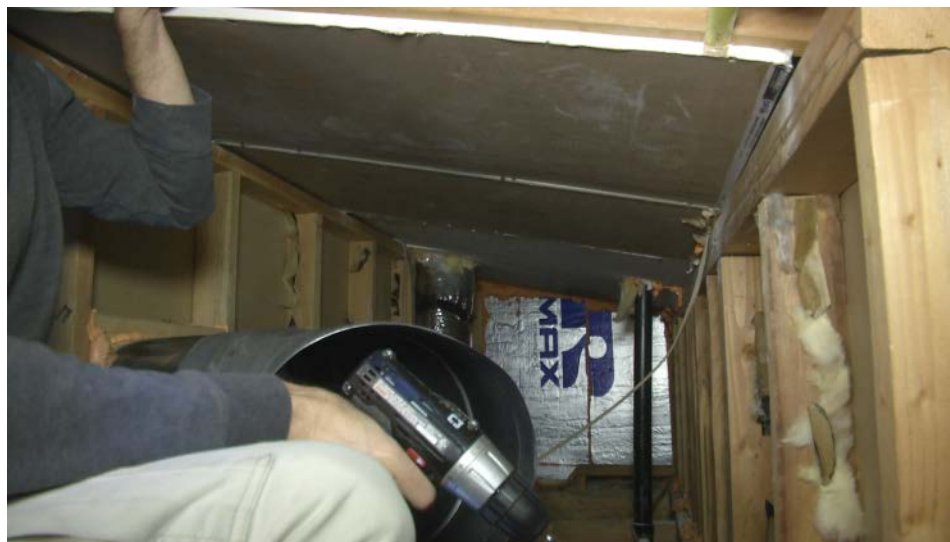
Figure 29. Pressure boundary being moved up to the bottom of the scissor trusses to allow ducts to remain within the building envelope
