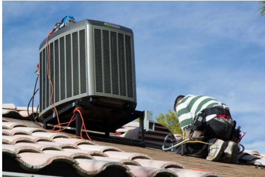
Figure 22. New outdoor heat pump unit being installed at the Sierra Hills home
