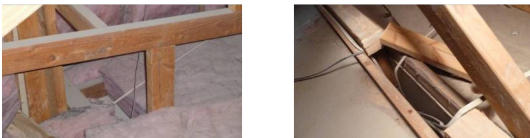
Figure 4. Top plate of interior walls cut out for electrical runs into partition walls
