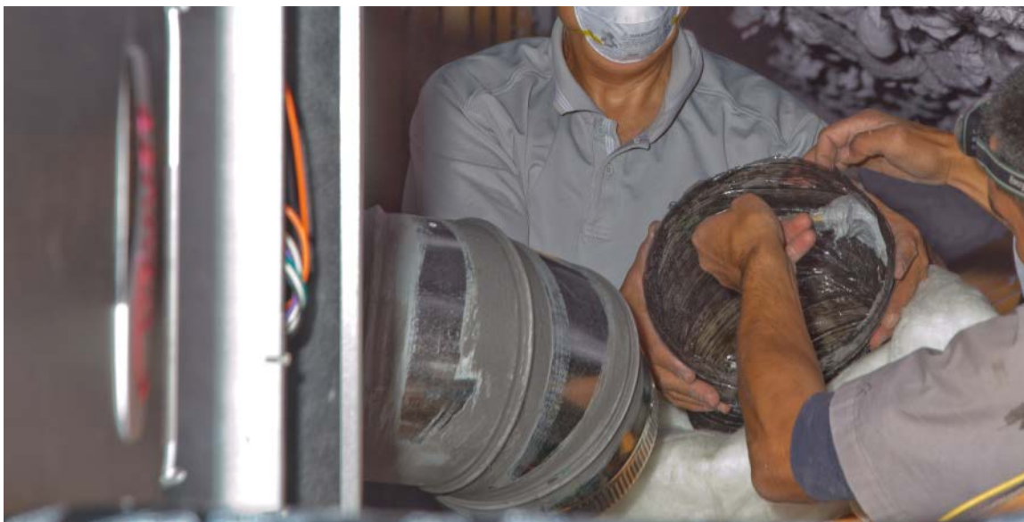
Figure 26. Mastic being applied to inside of flexduct jacket before being slipped over and secured to a branch takeoff elbow with compression bands
