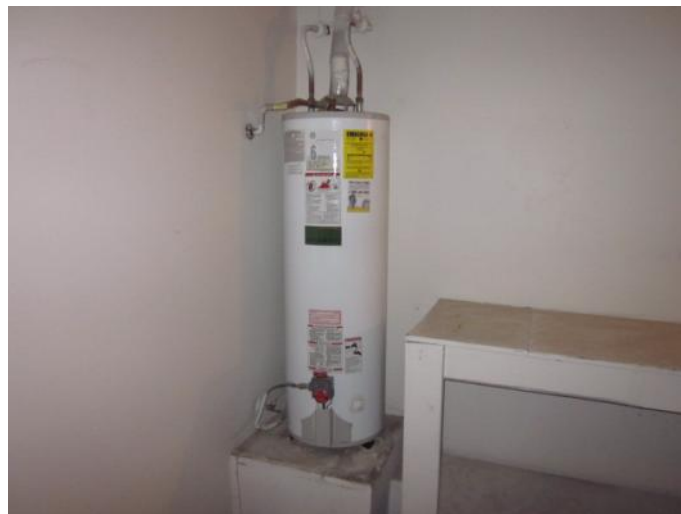
Figure 16. Atmospheric water heater located in the garage of the Sierra Hills home (Image courtesy of Building Media, Inc.)
