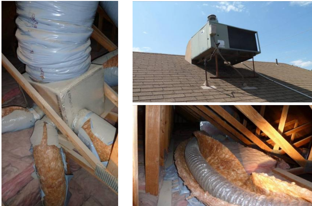
Figure 8. From left clockwise: supply plenum located in the vented attic, roof-mounted packaged furnace/AC, and insulation unwrapping from flex duct because the exterior vapor barrier had deteriorated
