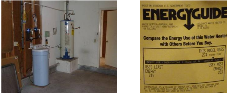
Figure 9. Atmospheric gas water heater located in the attached garage
