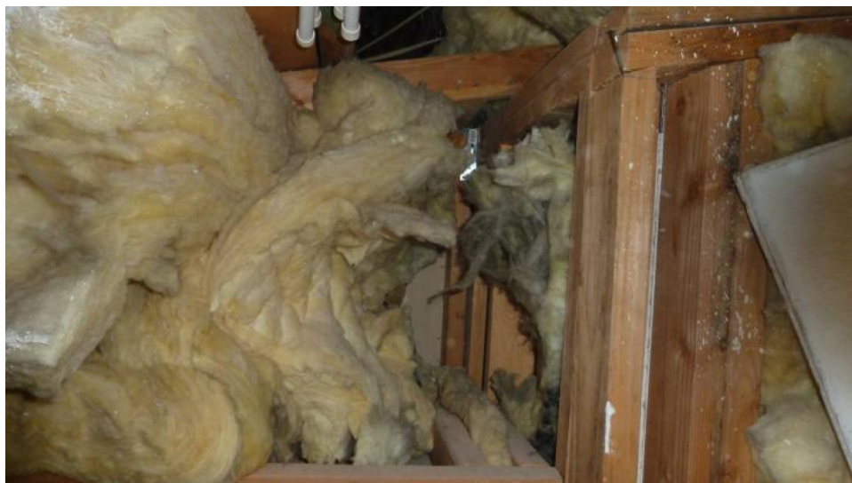
Figure 13. Poor insulating of partially vaulted ceiling kneewalls (Image courtesy of Building Media, Inc.)
