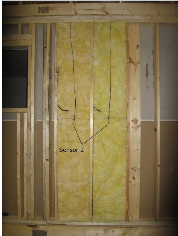
Figure 4: Sensor 2, both bays, prior to installing exterior sheathing.
