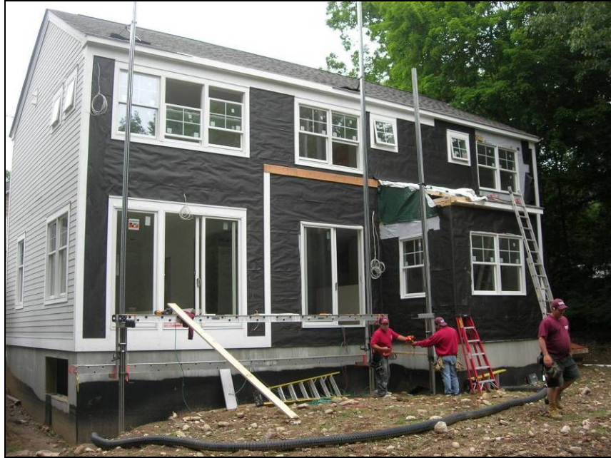
Figure 2: South side prior to installing fiber cement siding.
