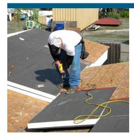
To add insulation while preserving the home's open-beam ceiling, workers place 6 inches of rigid R-38 urethane foam panels on top of the roof deck. SMUD's Mike Keesee said it was an unusual yet successful approach to insulating a residential building.
