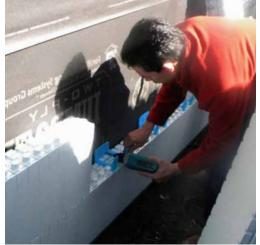
Workers place the first row of R-18 expanded polystyrene panels on a galvanized steel starting track. The foam panels insulate the home and give it a fresh new exterior.
