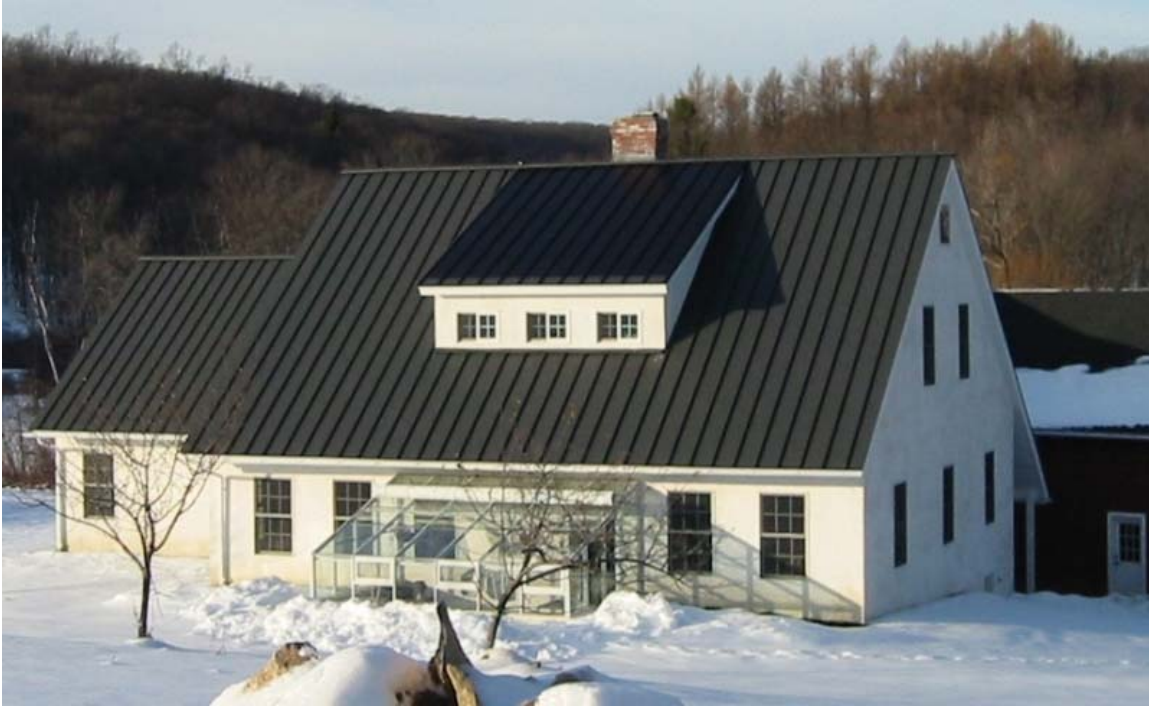
Figure 1. The home in Litchfield, CT with roof-integrated solar thermal and electric systems.
