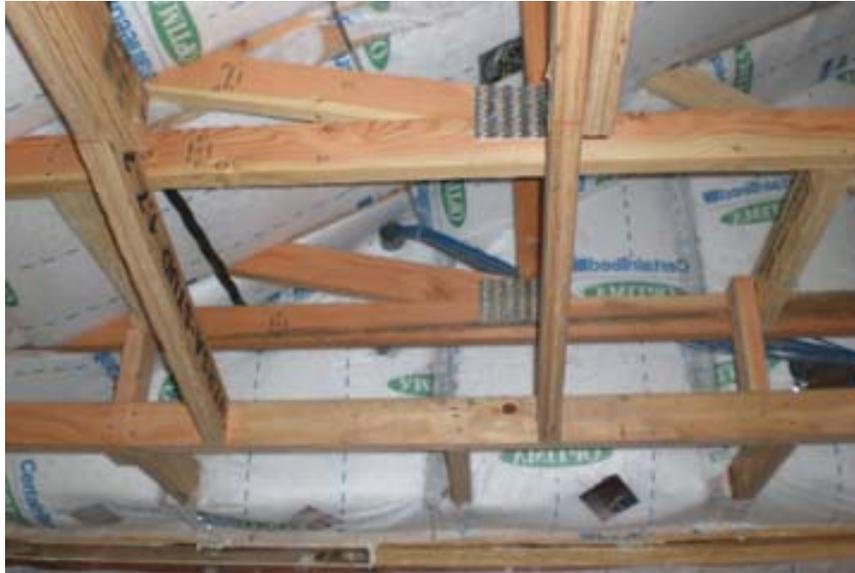
**Figure 6: Netted blown insulation at roof and kneewall**
