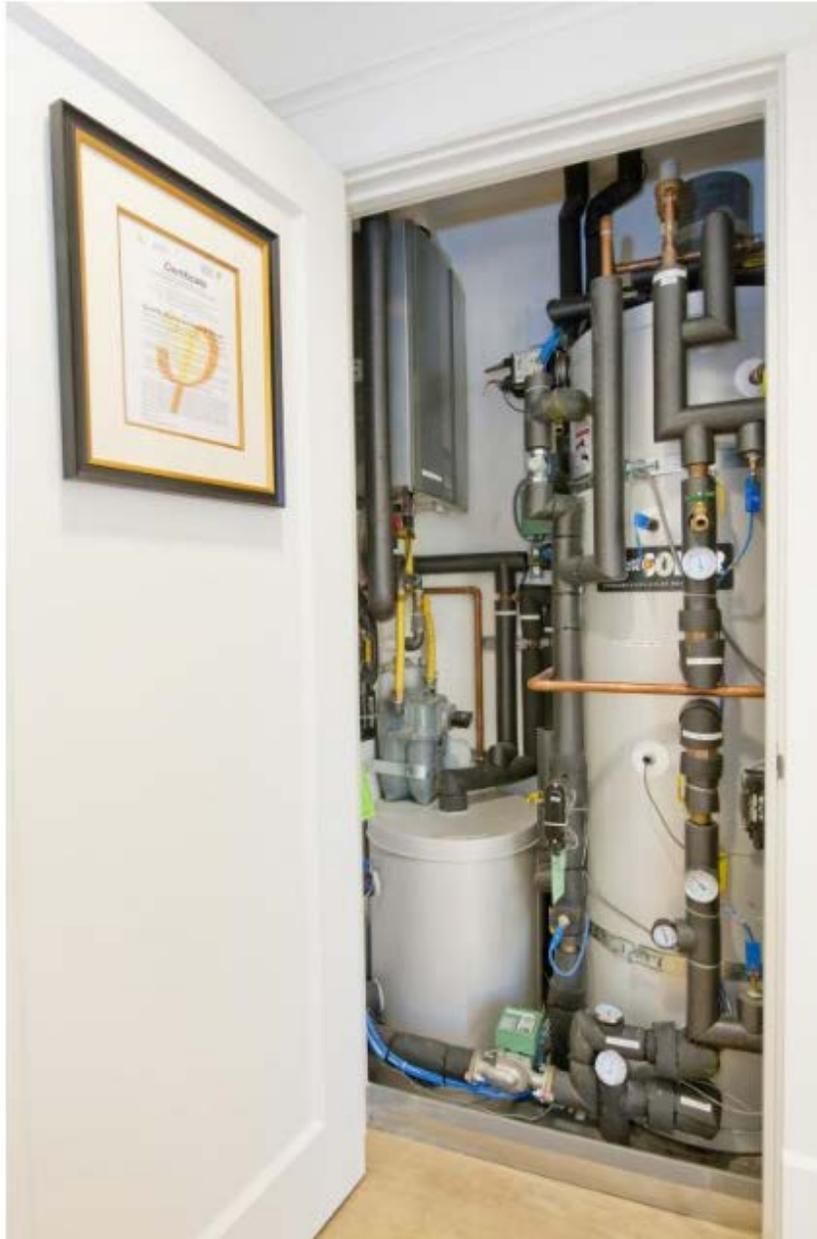
**Figure 8. Mechanical closet containing solar thermal storage system and tankless water heater**
