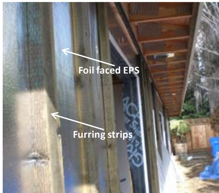
Figure 5. Exterior wall showing foil-faced EPS and furring for siding
