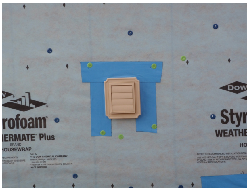
Figure 48. Photo of Properly Sealed Wall Penetration
