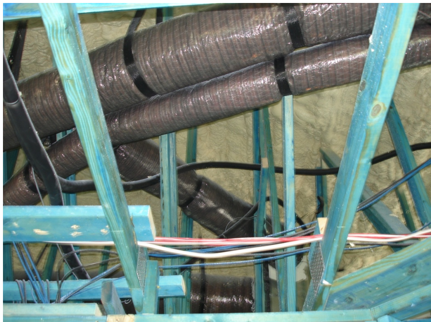
Figure 27. Photo of Attic Insulation Under Roof Deck
