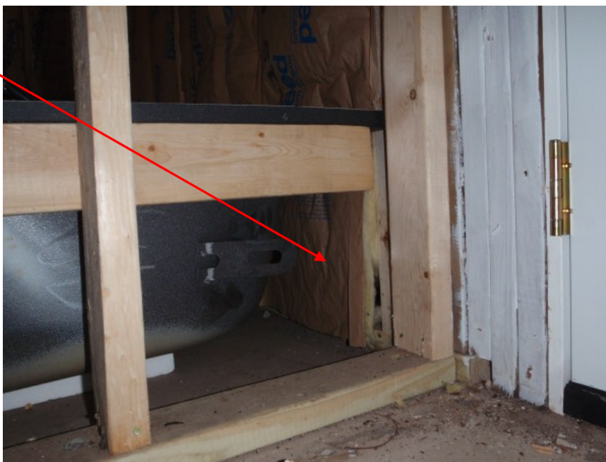
Figure 12. Photo of Missing Draftstopping
