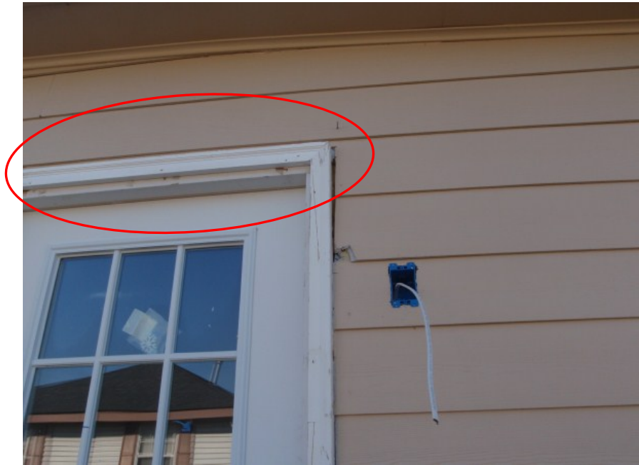
Figure 42. Photo of Missing Drip Cap at Door Head
