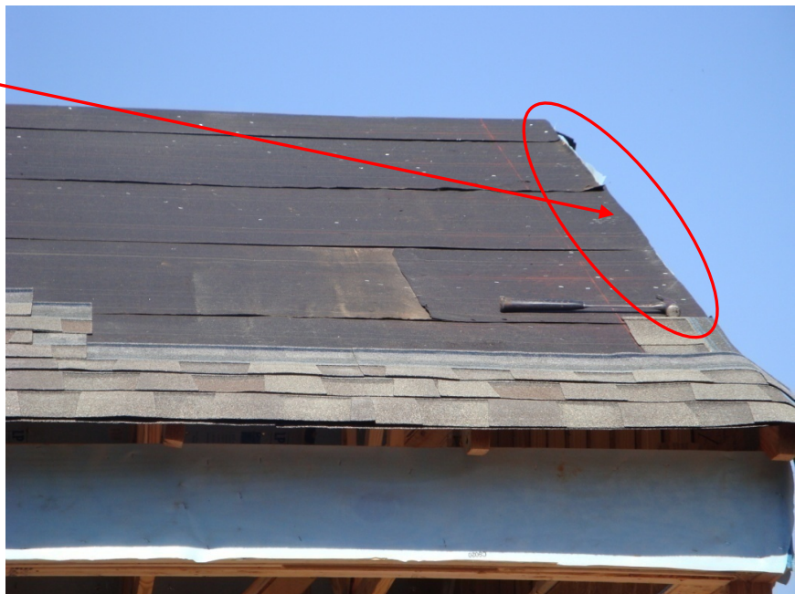
Figure 54. Photo of Proper Underlayment Installation at Roof Edge
