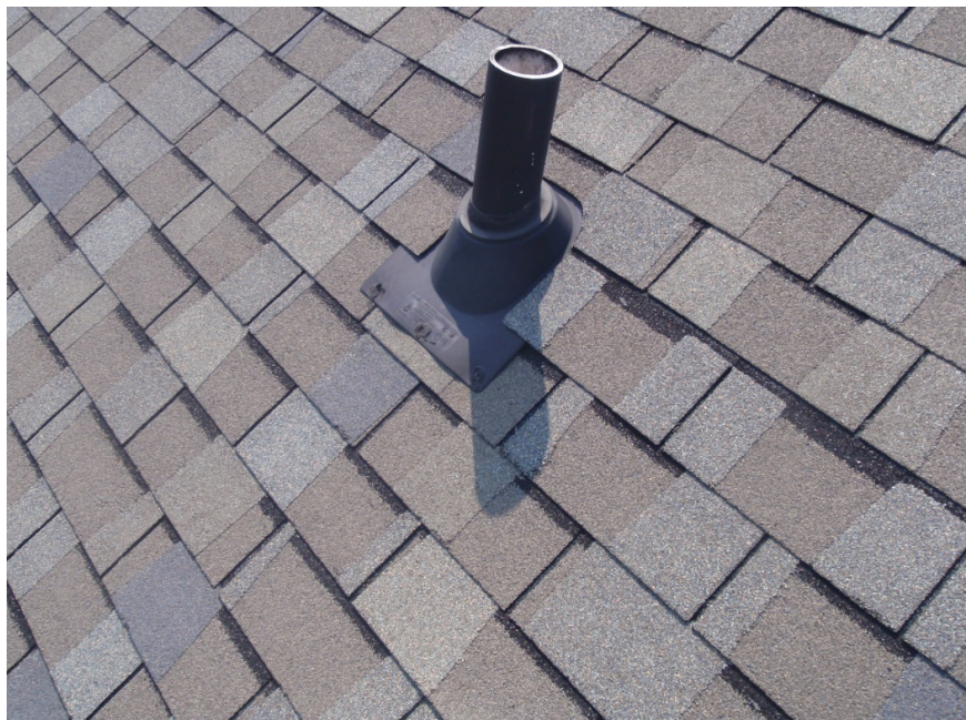
Figure 52. Photo of Proper Roof Boot Installation
