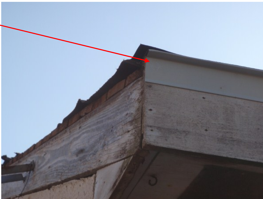
Figure 50. Photo of Properly Installed Drip Edge
