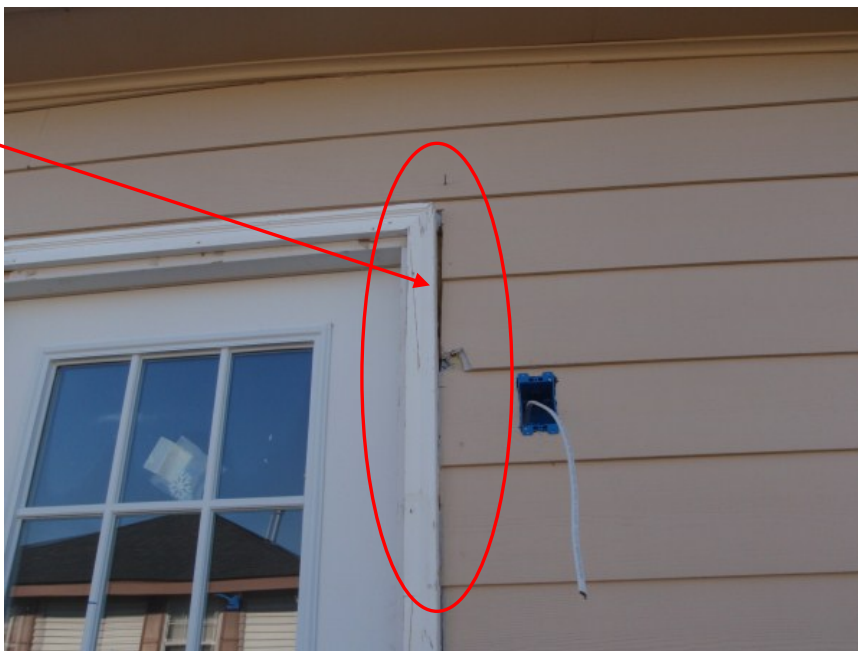
Figure 40. Photo of Missing Door Flashing
