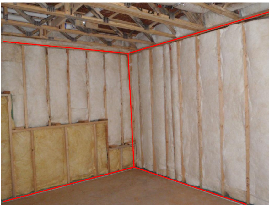
Figure 15. Illustration of Continuous Drywall Application
