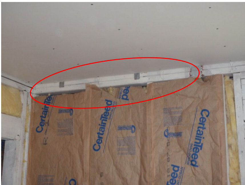
Figure 28. Photo of Short Kraft Faced Fiberglass Batts
