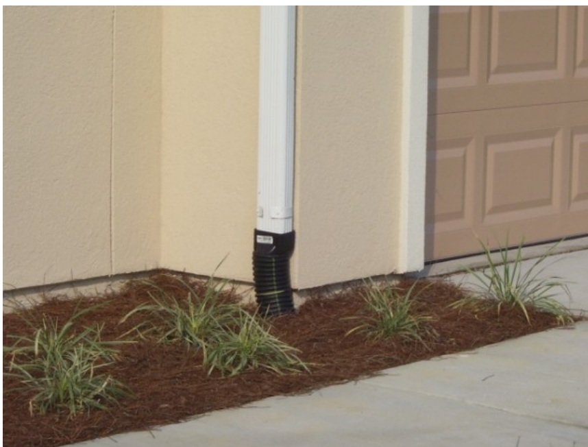
Figure 56. Photo of Effective Roof Drainage Discharge
