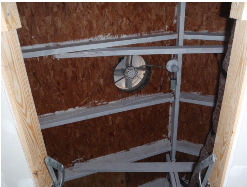
Figure 36. Photo of Attic Exhaust Fan
