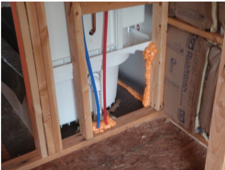
Figure 13. Photo of Proper Draftstopping
