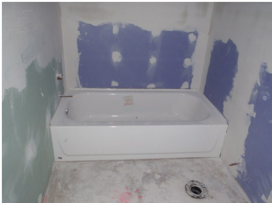
Figure 63. Photo of Proper Back Board Installation
