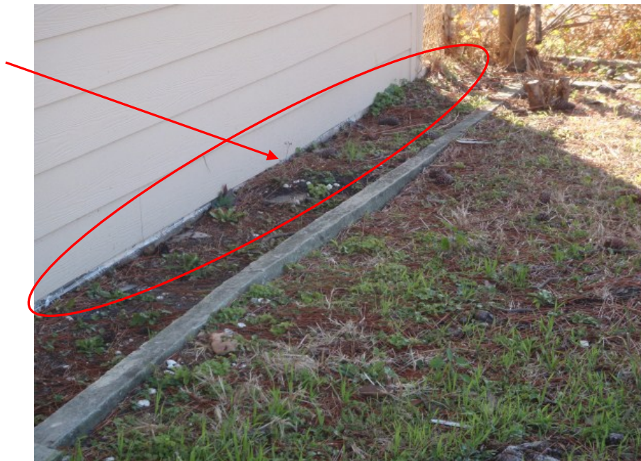
Figure 57. Photo of Insufficient Grade Separation
