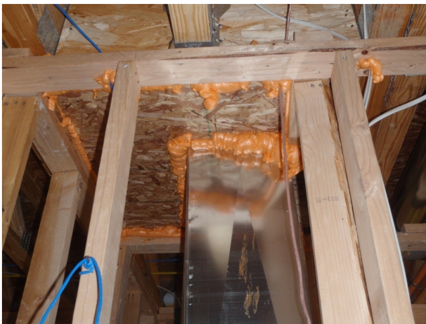
Figure 11. Photo of Sealed Mechanical Chase Lid
