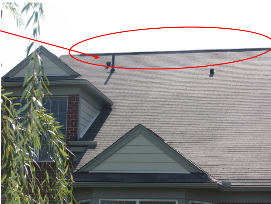
Figure 37. Photo Attic Ridge Venting
