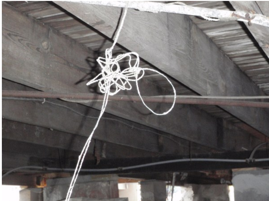
Figure 22. Photo of Uninsulated Raised Floors
