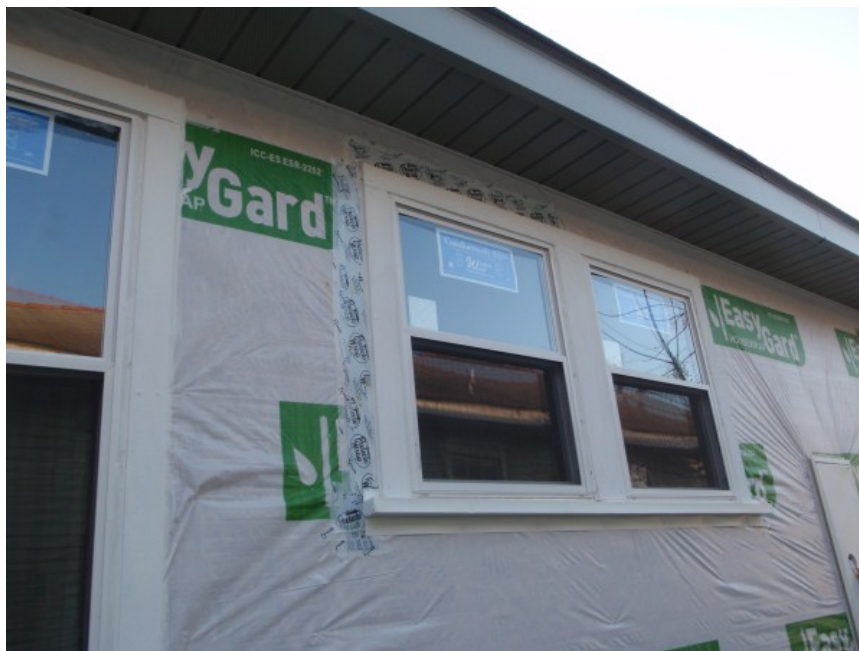
Figure 45. Photo of Mis-lapped Window Flashing
