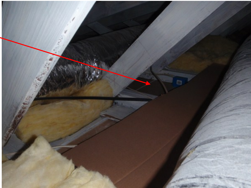
Figure 26. Photo of Missing Attic Insulation
