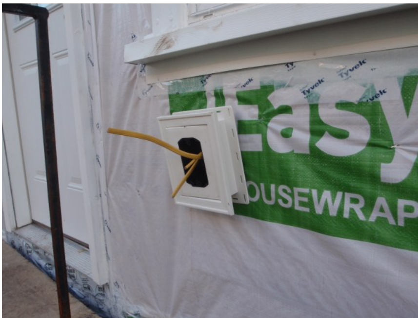
Figure 47. Photo of Unsealed Wall Penetration
