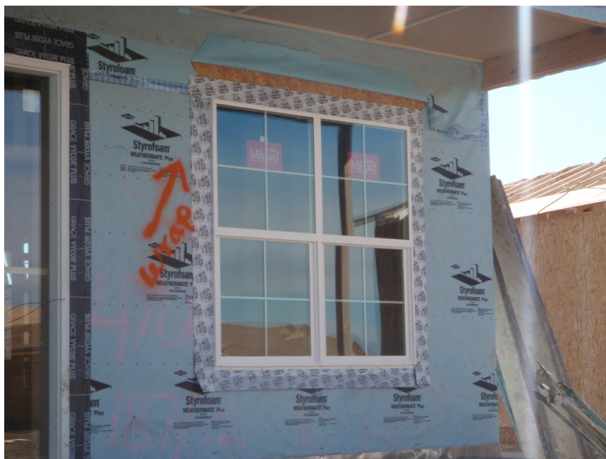
Figure 46. Photo of Proper Window Flashing Installation
