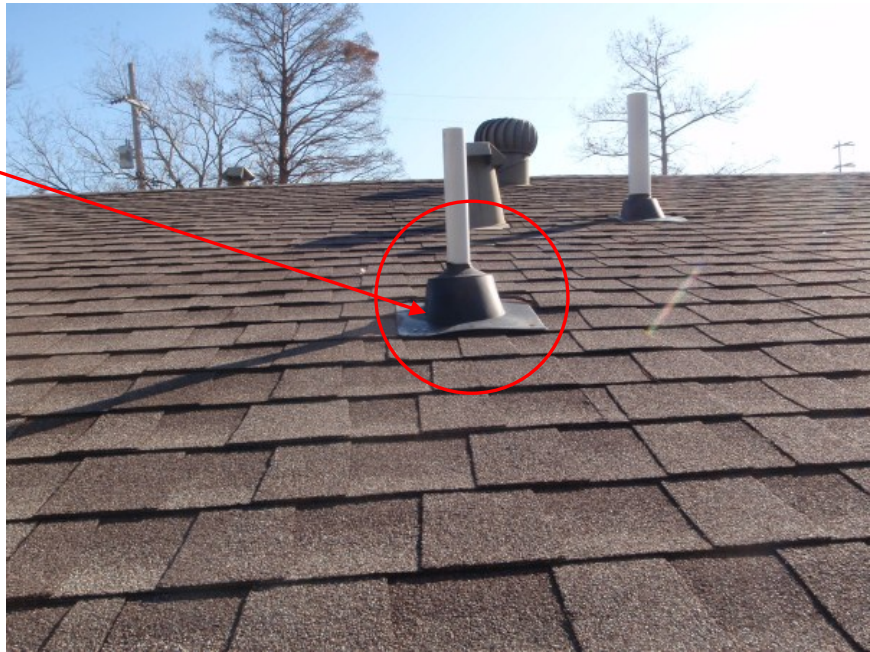
Figure 51. Photo of Improper Roof Boot Installation
