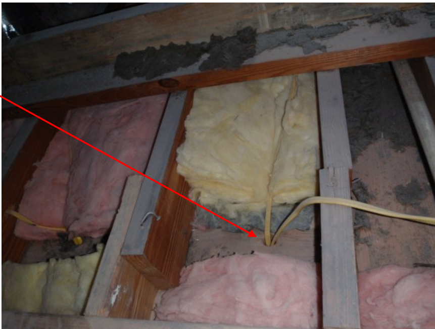
Figure 24. Photo of Missing Attic Insulation at Ceiling
