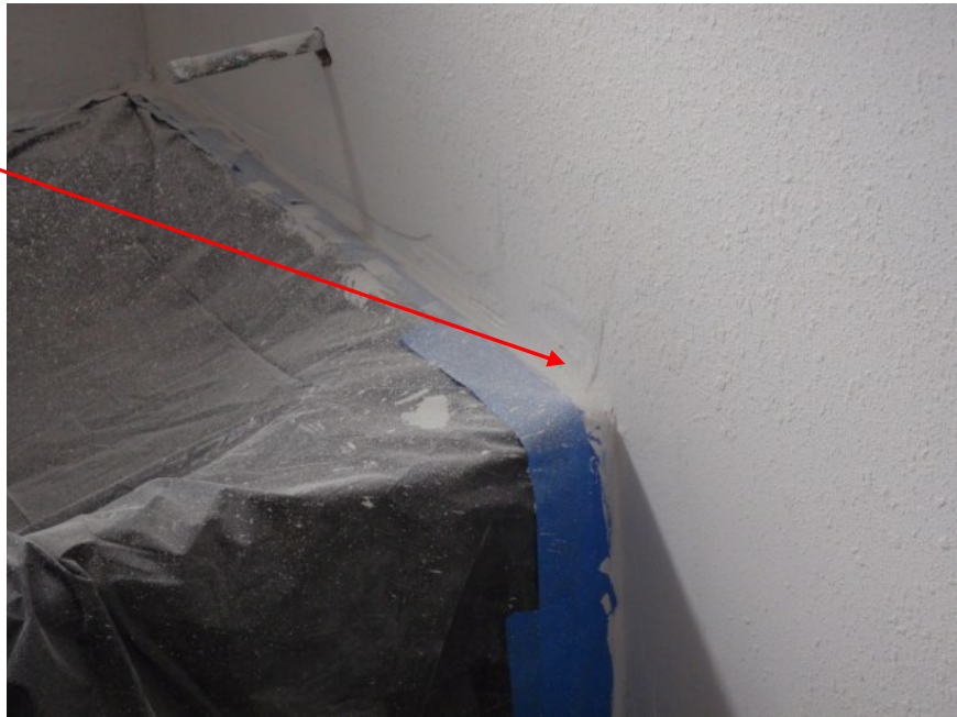
Figure 62. Photo of Improper Backer Board Installation
