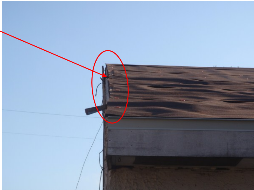
Figure 53. Photo of Insufficient Underlayment at Roof Edge
