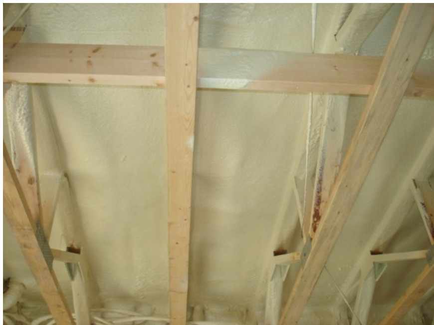
Figure 23. Photo of Closed Cell Foam Under Floor Decking
