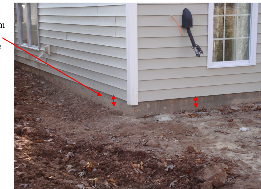
Figure 58. Photo of Adequate Grade Separation
