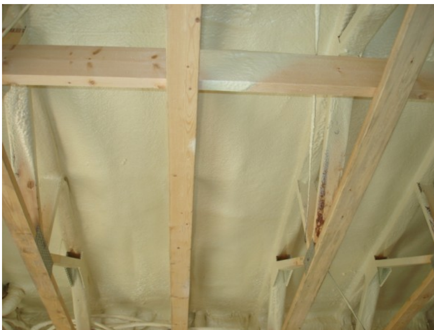
Figure 19. Photo of Closed Cell Foam Under Floor Decking
