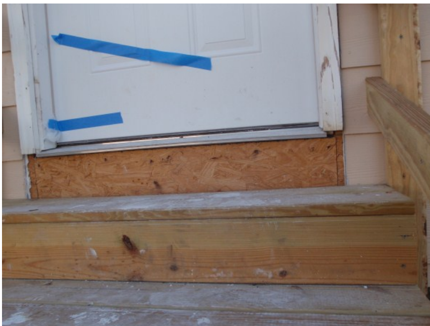
Figure 38. Photo of Missing Door Flashing
