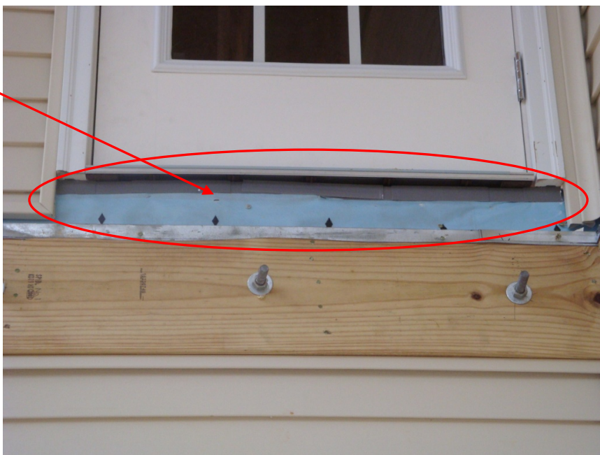
Figure 39. Photo of Proper Door Sill Flashing Installation
