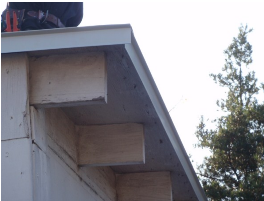
Figure 49. Photo of Improperly Installed Drip Edge
