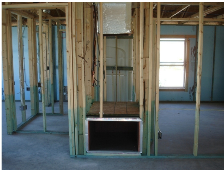
Figure 31. Photo of Sealed Return
