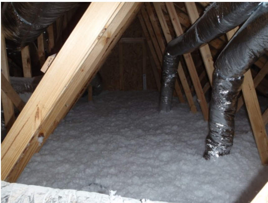
Figure 25. Photo of Well Insulated Attic at Ceiling
