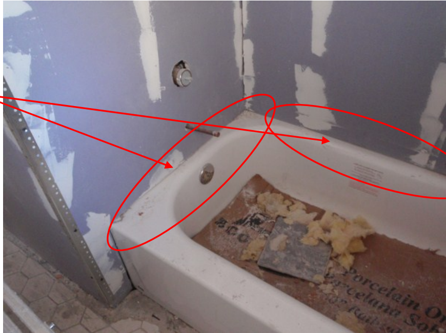
Figure 59. Photo of Insufficient Flashing Surrounding Tub
