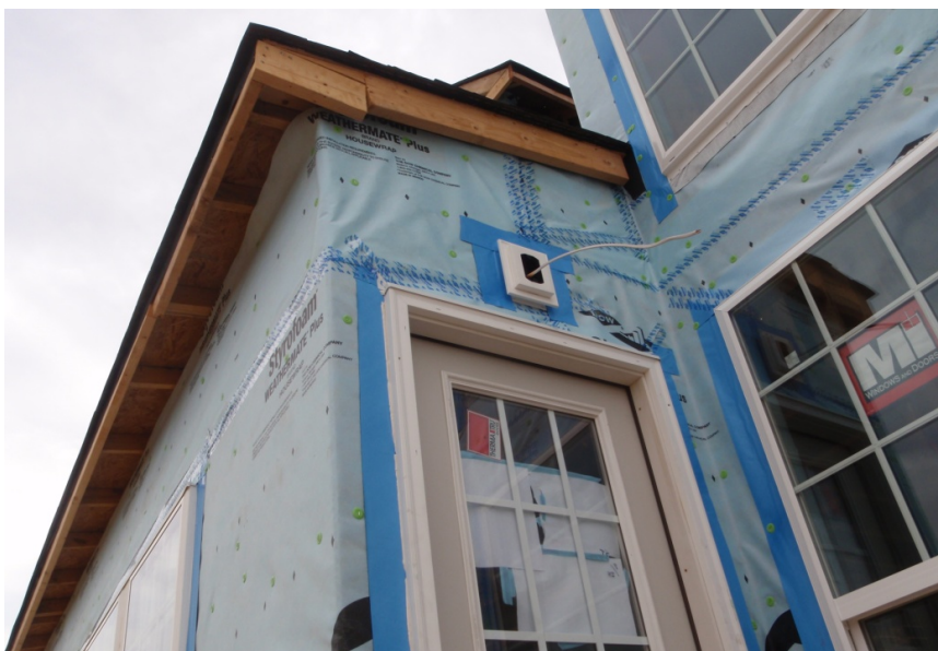
Figure 41. Photo of Proper Door Flashing Installation
