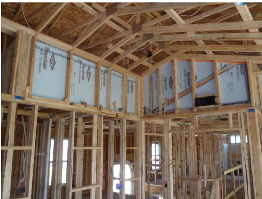
Figure 21. Photo of Properly Sheathed Attic Kneewalls
