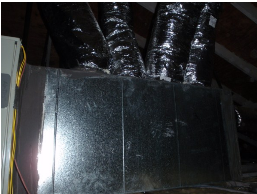
Figure 32. Photo of Identically Sized Ducts
