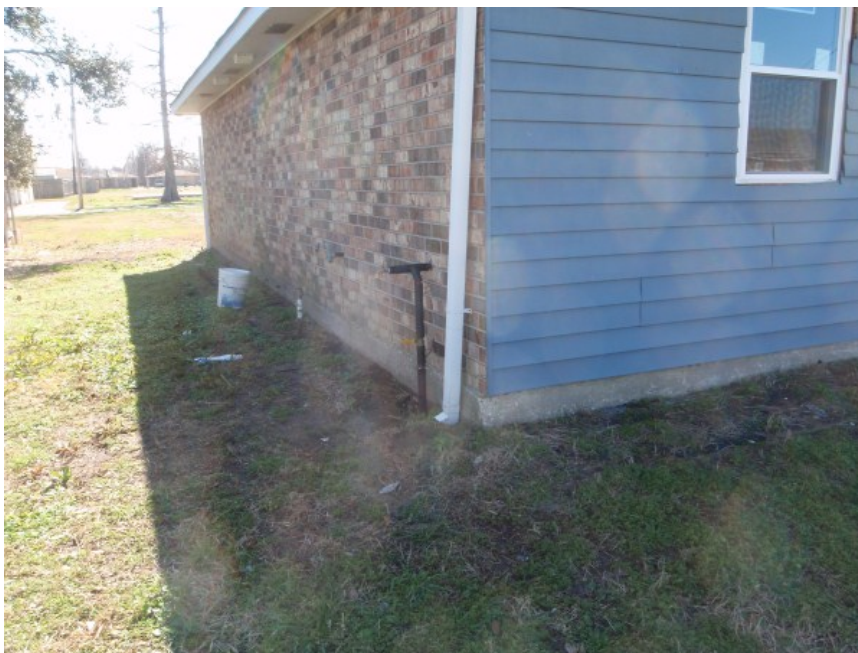
Figure 55. Photo of Downspout Discharge Against Foundation
