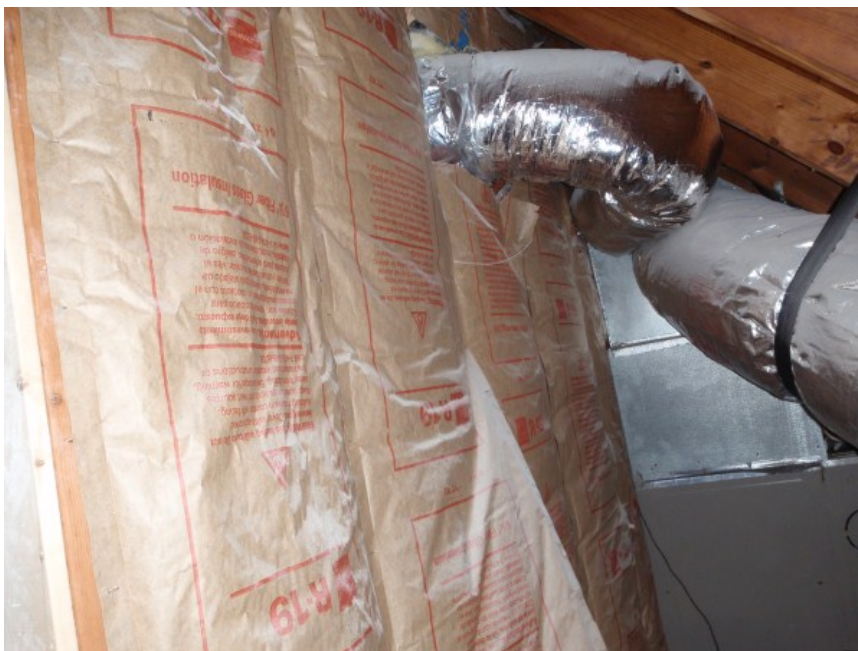
Figure 20. Photo of Unsheathed Attic Knee Walls
