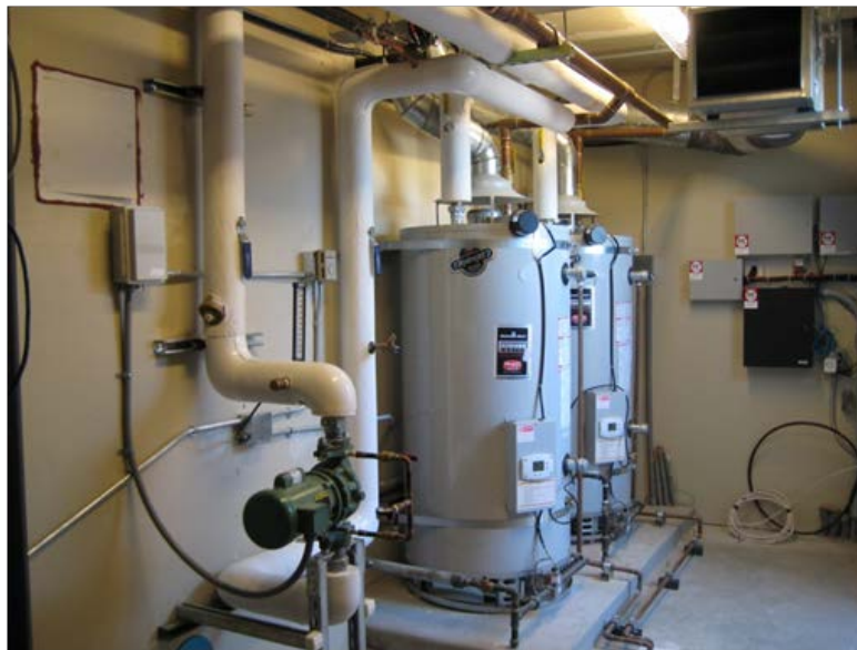
Figure 8. Central system utilizing two large storage water heaters
