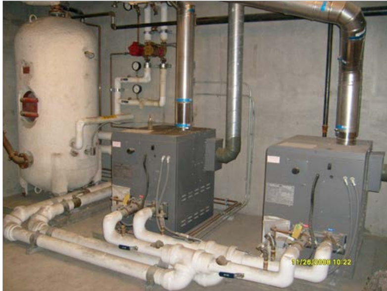
Figure 7. Central system utilizing two circulating boilers with storage tank
