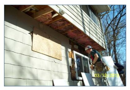
Figure 3. Typical cantilevered floor area depicting issues leading to performance problems
