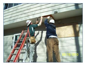
Figure 8. Cantilevered floor blocking, air sealing, and insulation
