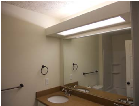
Figure 10. Light soffit.
