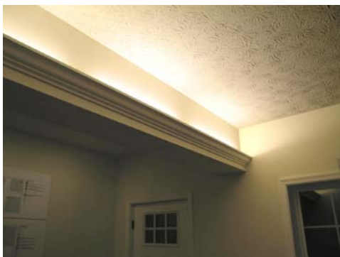
Figure 4. Architecturally integrated light cove.
