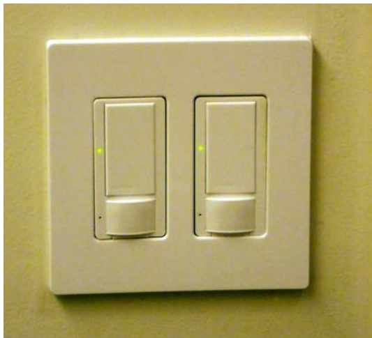
Figure 93. Manual on/automatic off control.
