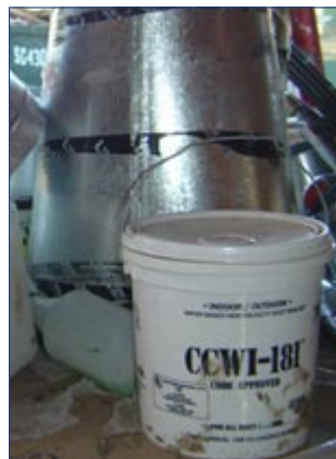
Careful duct sealing with mastic helps improve comfort and energy efficiency at low cost.
