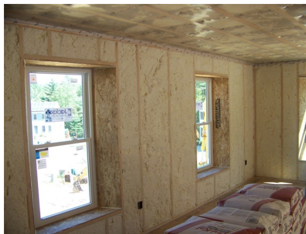
Figure 44. Typical installation of ½ lb/ft 3 spray foam in double-stud walls
