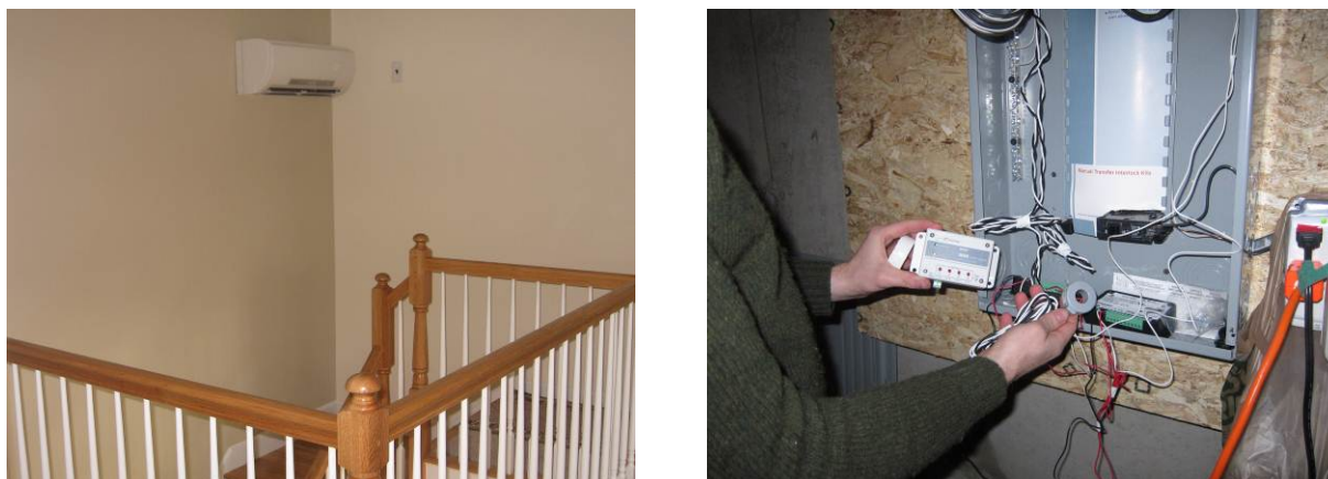
Figure 22. (L) Upstairs mini-split at Easthampton; (R) Watt-hour meter at Devens
