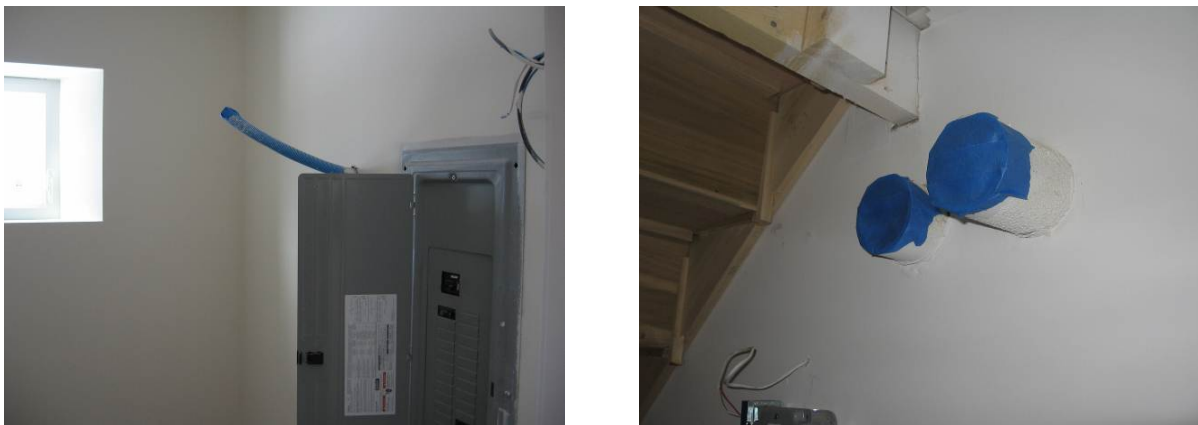
Figure 18. (L) PV inverter connection; (R) tankless water heater intake and exhaust vent
