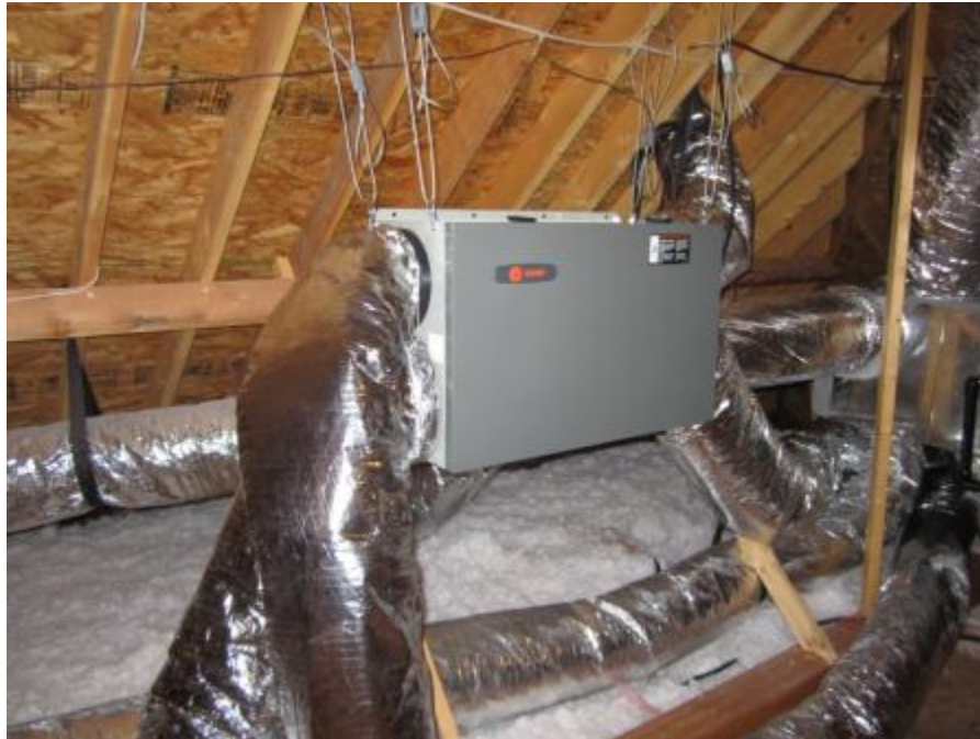
Figure 7. Energy recovery ventilator (ERV) installed in House 1 to match that of House 2
