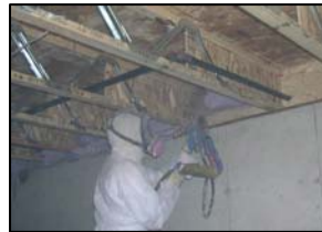
Foaming the rim joist
