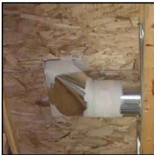
Reducing leakage at the boots
