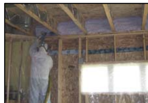
Corbond at the first floor band joist
