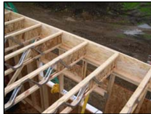
Inline Space Joist floor system
