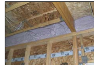
Foam tightly seals penetrations
