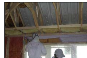
Insulated window headers
