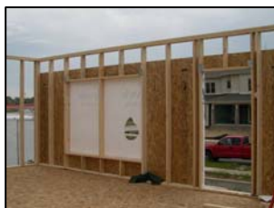
24” OC, window header hangers, double top plate
