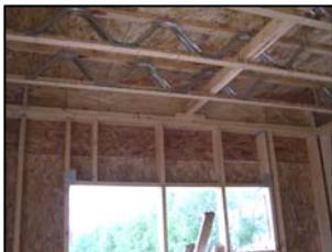
Window header in floor system
