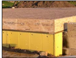
Foundation Insulation Detail
