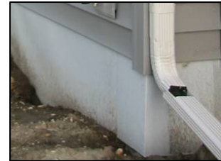
Foundation Flashing Detail
