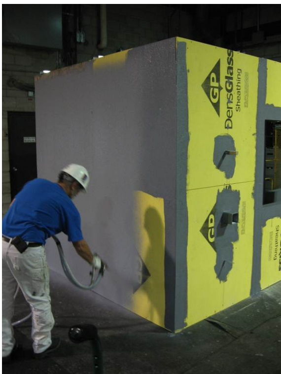
Figure 13. Spray applied liquid applied barrier
