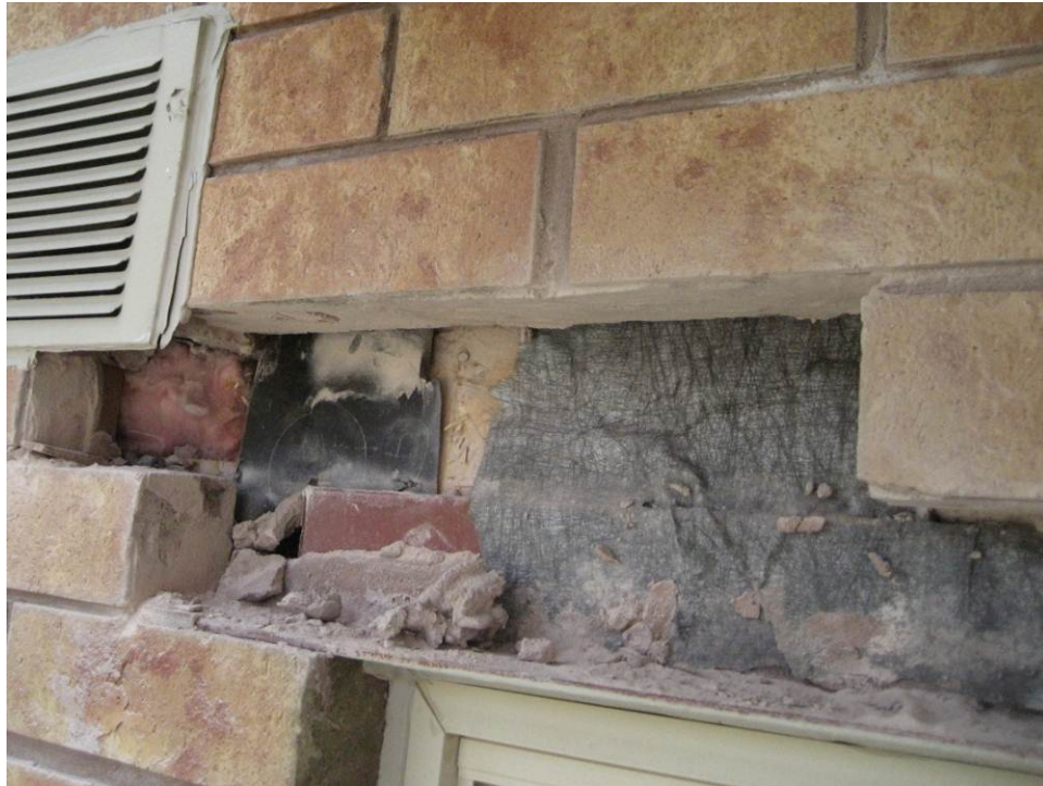
Figure 3. Intrusive investigation of the water management details. Note the poor execution of the mechanical penetration, the gap in sheathing membrane continuity, which will allow water and air leakage, and the bonding of the mortar to the membrane.
