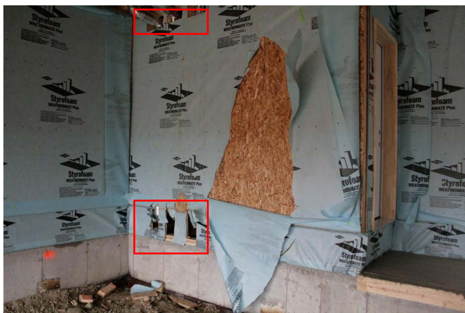
Figure 1. House wrap installation in new construction. The large tear will likely be fixed before construction continues — see one manufacturer’s instructions in Figure 2. The smaller deficiencies (highlighted) are often not addressed.
