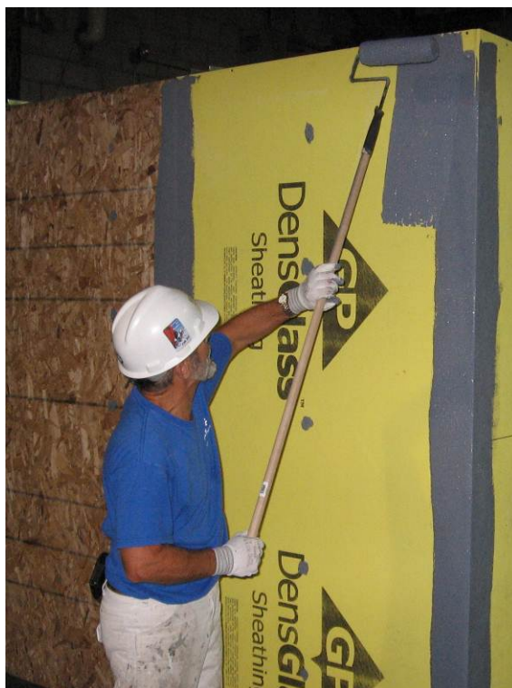
Figure 14. Roller applied liquid applied barrier
