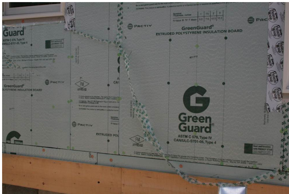
Figure 6. Taped exterior insulation drainage plane
