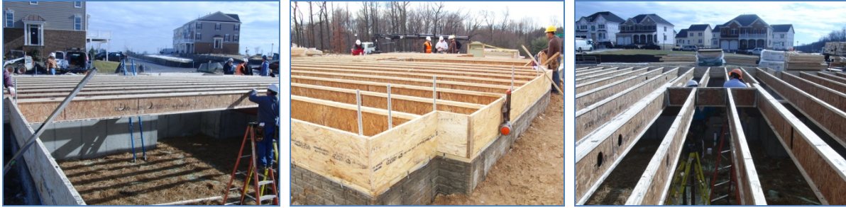
Figure 4. Floor framing
