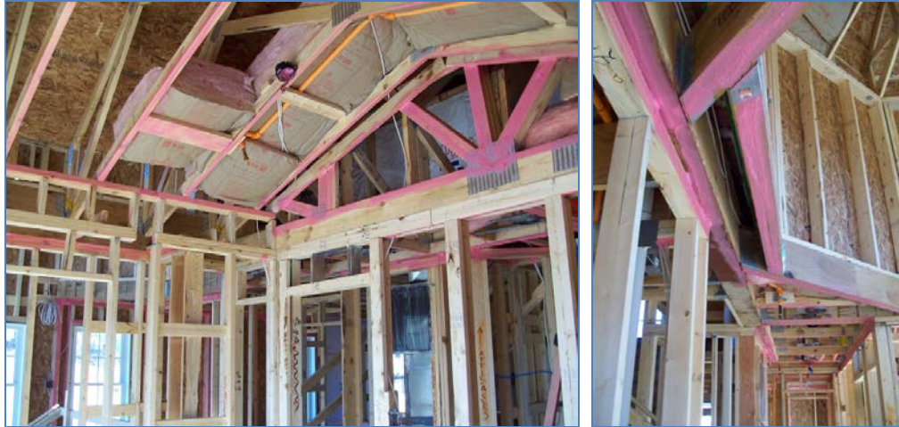
Figure 9. Complex thermal air boundary (2 of 3)
