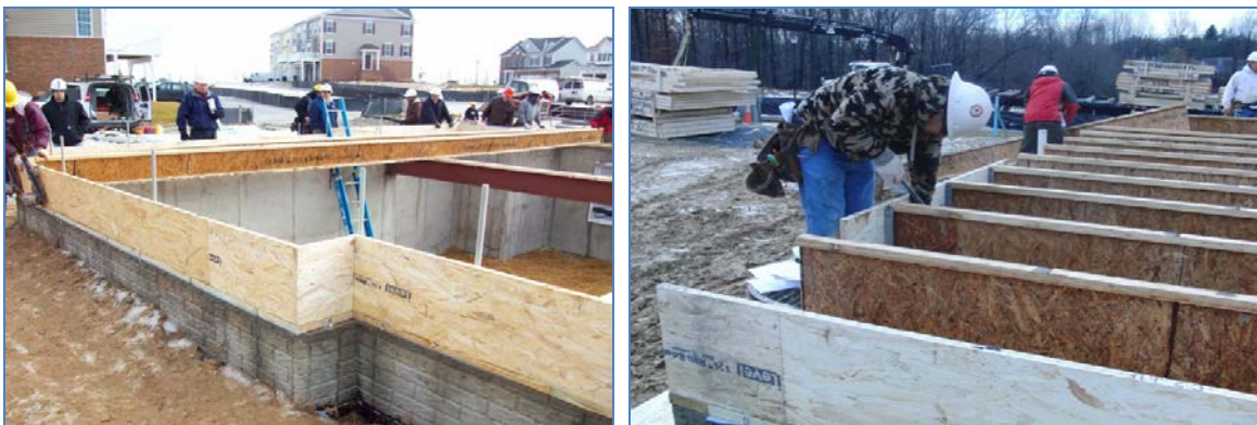
Figure 17. Floor framing
