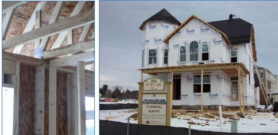
Figure 7. Raised heel truss with increased overhang at eaves
