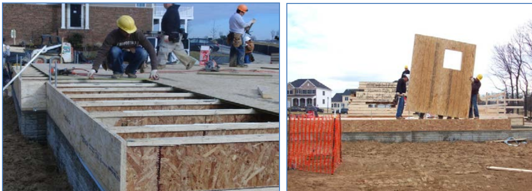
Figure 18. Floor framing and wall panels
