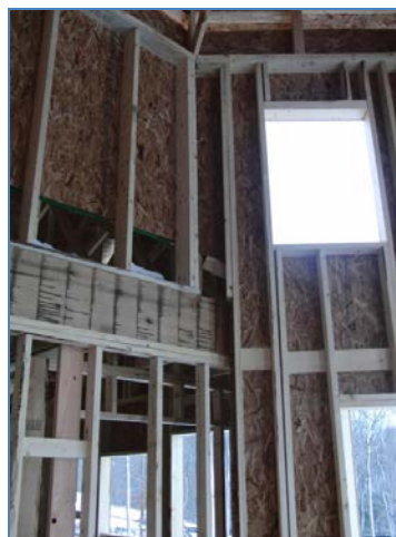
Figure 8. Complex thermal air boundary (1 of 3)
