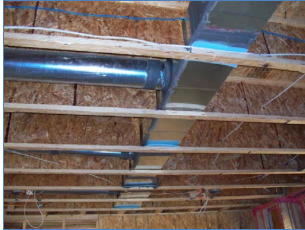
Figure 15. HVAC supply trunk installed in second-floor framing
