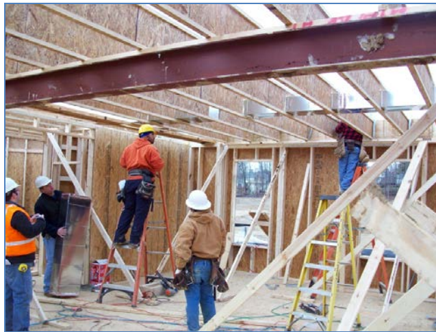
Figure 24. Installing HVAC trunk through floor joists
