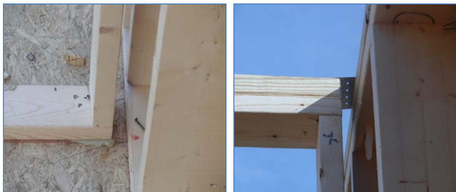
Figure 6. Continuous drywall method
