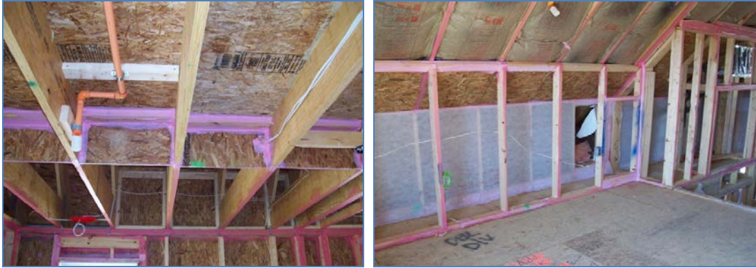
Figure 21. Air sealing at blocking below third-floor knee wall and knee walls
