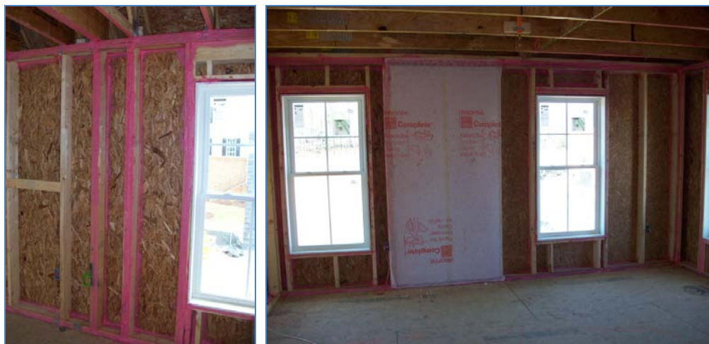
Figure 11. Air sealing
