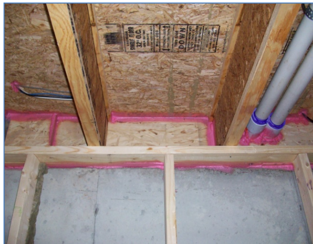
Figure 22. Air sealing at basement rim area
