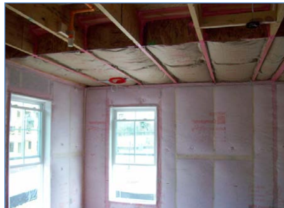
Figure 13. Wall and attic insulation
