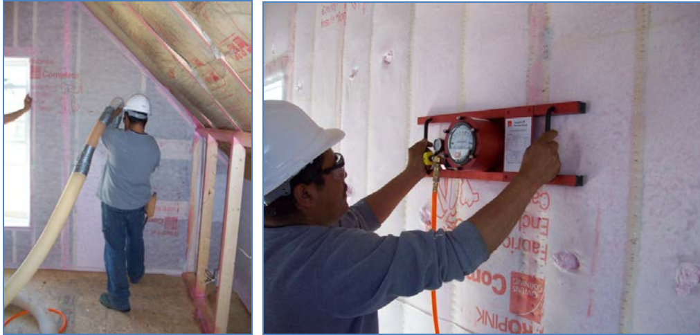
Figure 23. Installing wall cavity blown insulation and checking density
