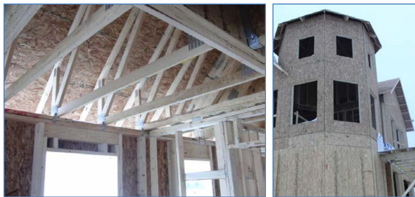
Figure 20. Wall panels and trusses
