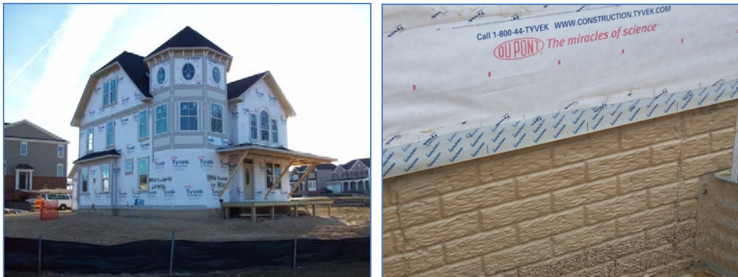
Figure 12. House wrap installed as air barrier
