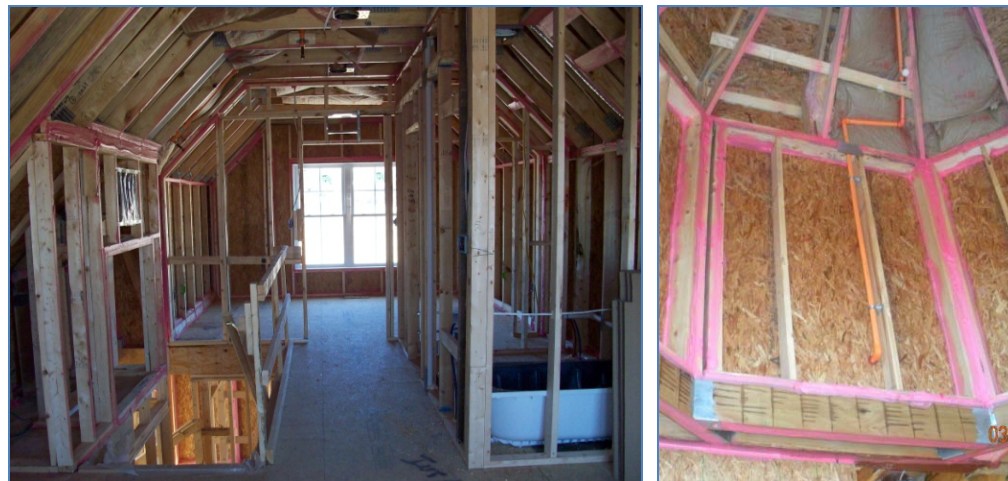
Figure 10. Complex thermal air boundary (3 of 3)
