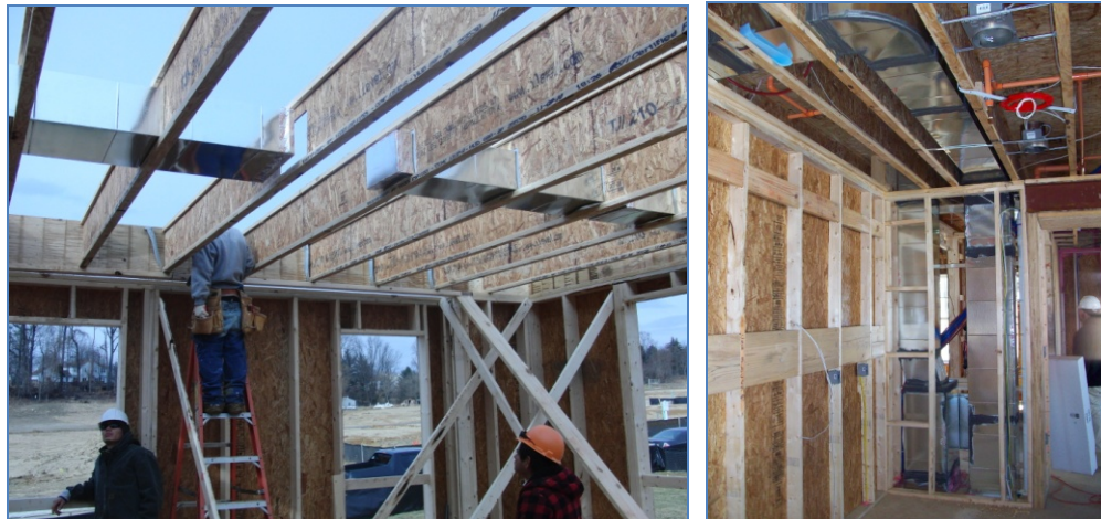
Figure 3. Supply trunk through floor joists and central duct chase
