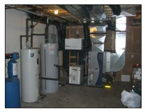
CARB extensively monitored this GSHP system. CARB coordinated with the plumber to have thermowells installed at fluid temperature measurement points to ensure accuracy of these measurements. Inline flow meters were also installed.
