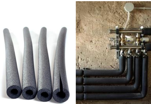
Figure 6-20: Typical Use of Piping Insulation
