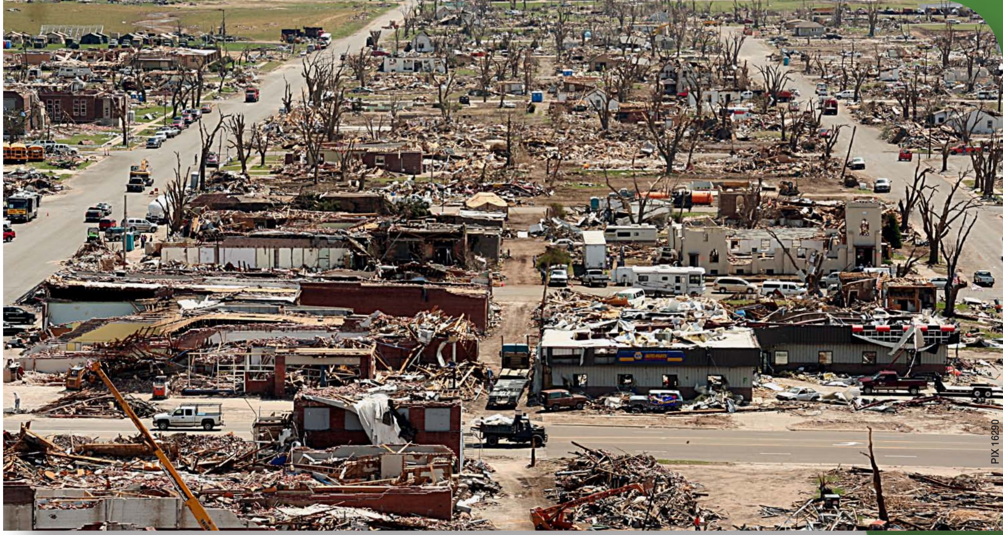
Courtesy of Federal Emergency Management Agency
