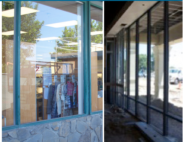
Original storefront windows with no thermal breaks (left) were replaced with new glazing providing thermal breaks and control of solar heat gain (right)
