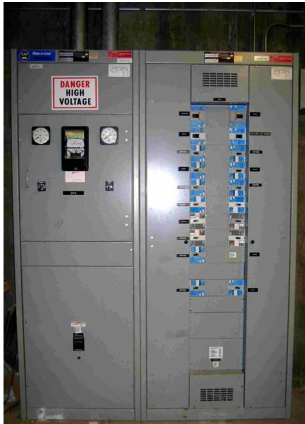
Figure 4.2. Building B - Distribution Panel with Three-Phase Lighting Riser Logger Installed in Right-Hand Compartment
