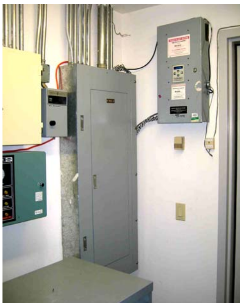
Figure 3.1. End Use Metering Logger. The box to the right of the control panel is one of two end use metering loggers used to measure current, power, and apparent power in Building A.
