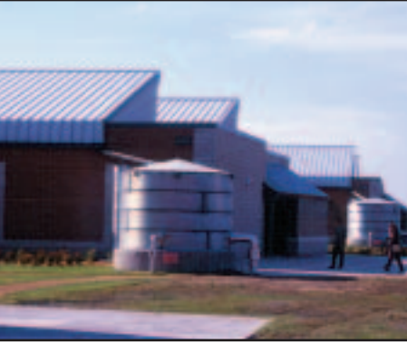
Using this cistern, the Roy Lee Walker Elementary School in McKinney, TX, harvests rainwater.
