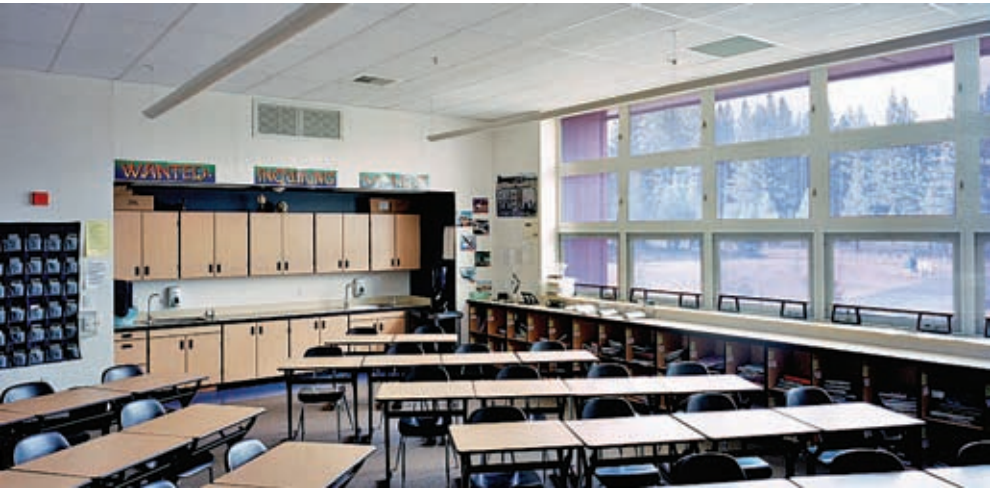
This typical classroom shows its daylighting and lighting systems. Light fixtures are 60 percent uplight and 40 percent downlight.
