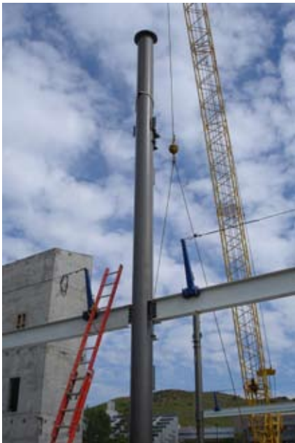
Reclaimed natural gas pipelines, which are repurposed as vertical structural columns are put in place at the construction site.
